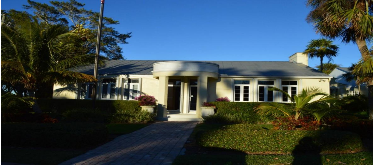
FIGURE 39. FEDERAL RECREATION BUILDING, 201 SW FLAGLER AVENUE
