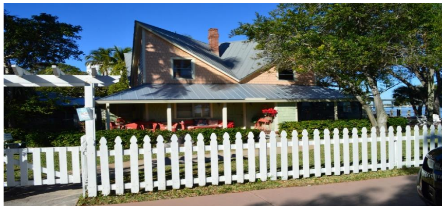
FIGURE 57. THE OWL HOUSE, 100 COLORADO AVENUE
