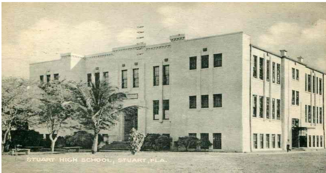
FIGURE 19. STUART HIGH SCHOOL, 500 SE OCEAN BLVD
