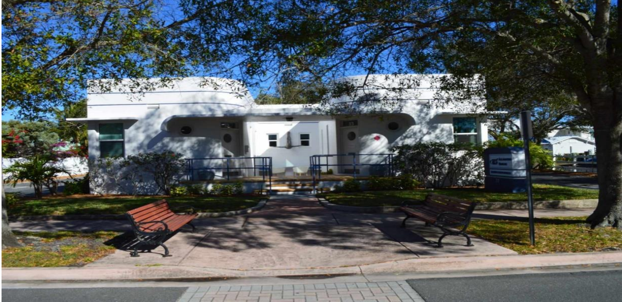
FIGURE 61. HIPSON OFFICE BUILDING, 31-33 SE OSCEOLA STREET
