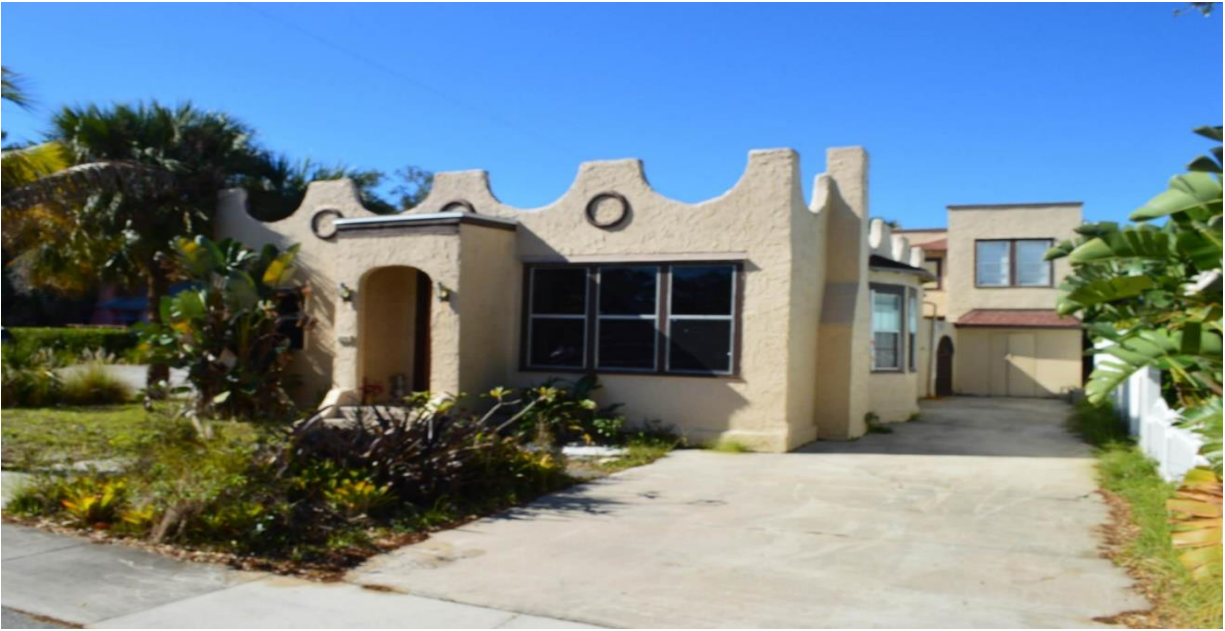
FIGURE 60. MISSION STYLE, 428 SW CAMDEN AVENUE
