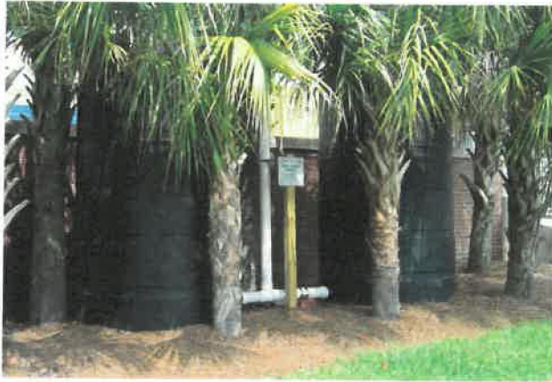
Two 1,550 gallon cisterns are used to harvest rainwater that has filtered through the Perry Construction Yard green roof at the University of Florida in Gainesville
