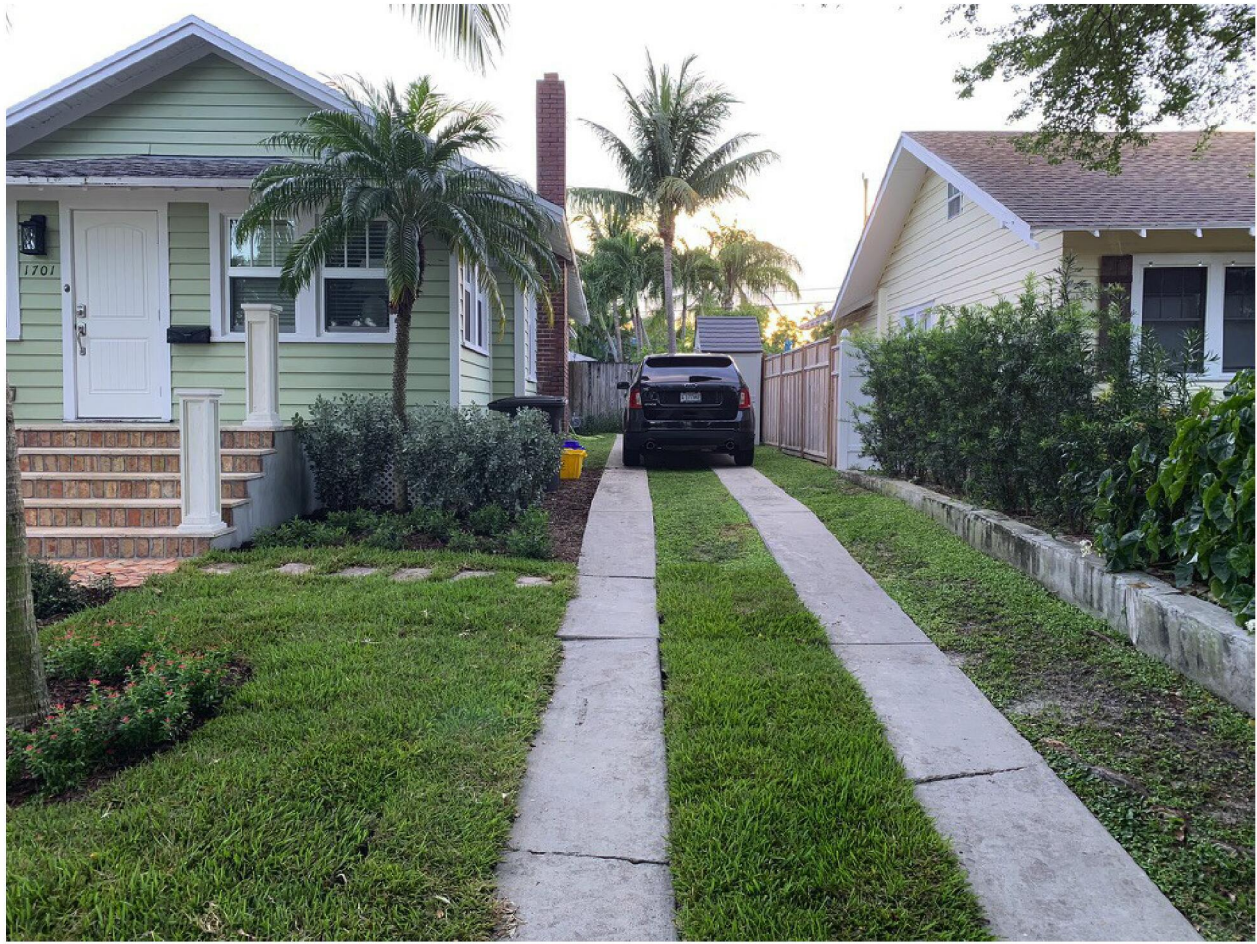
Figure 3: Ribbon Driveway with Concrete, Grandview Heights, West Palm Beach, FL
