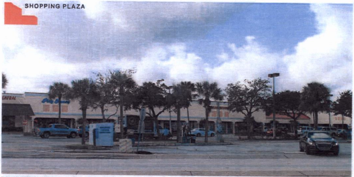
Figure 136 Image of site from Southwest Federal Highway.
