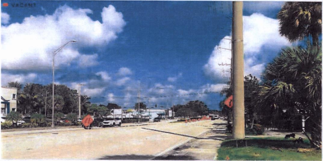
Figure 153 Image of site from Southwest Federal Highway.
