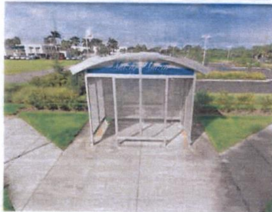
Figure 35 Typical Marty transit stop with shelter and bench. The pictured stop is at Indian River State College on Salerno Road.
