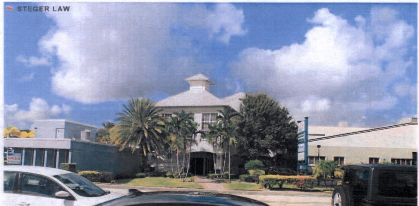
Figure 163 Image of site from Southwest Federal Highway.
