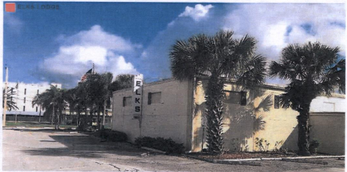
Figure 118 Image of site from South Kanner Highway.
