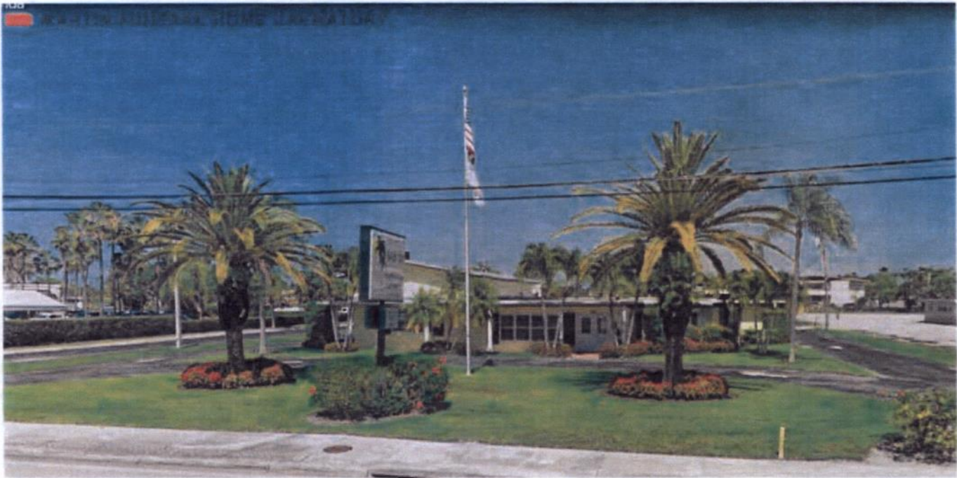
Figure 116 Image of site from South Kanner Highway.
