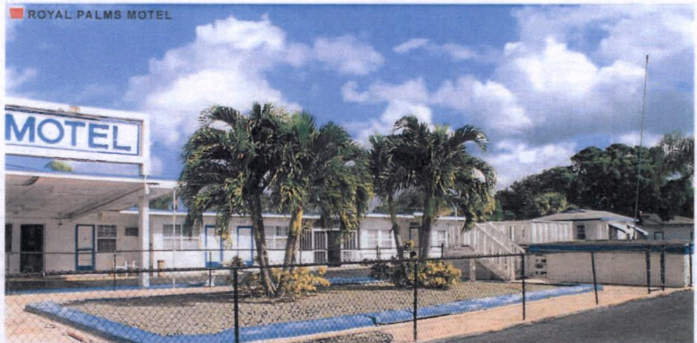
Figure 147 Image of site from Southwest Federal Highway.
