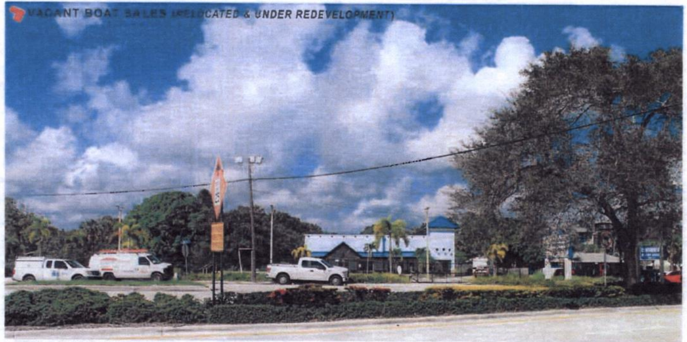
Figure 157 Image of site from Southwest Federal Highway.
