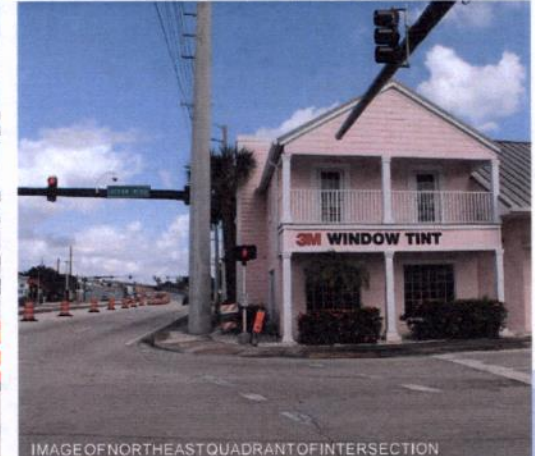
IMAGE OF NORTHEAST QUADRANT OF INTERSECTION
