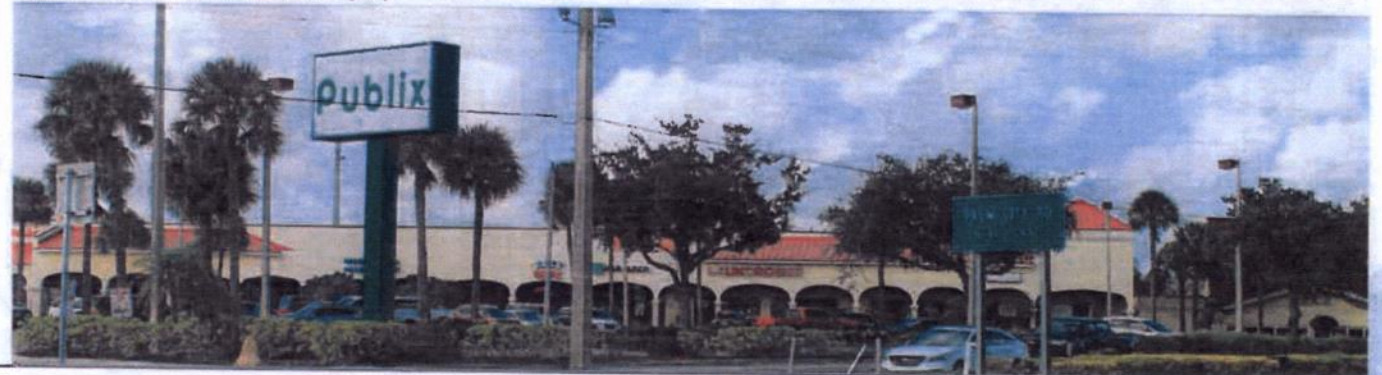
Figure 137 Image of site from Southwest Federal Highway.
