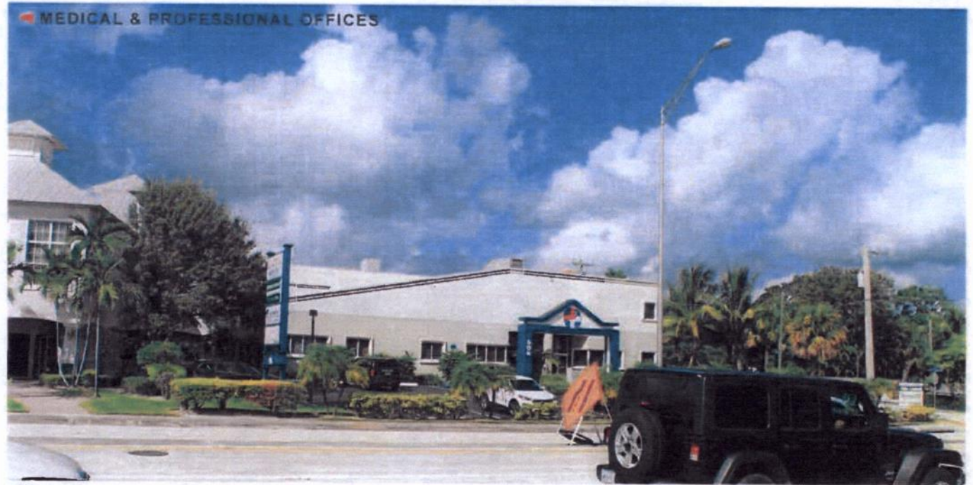
Figure 155 Image of site from Southwest Federal Highway.
