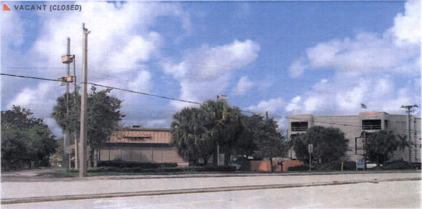
Figure 143 Image of site from Southwest Federal Highway.
