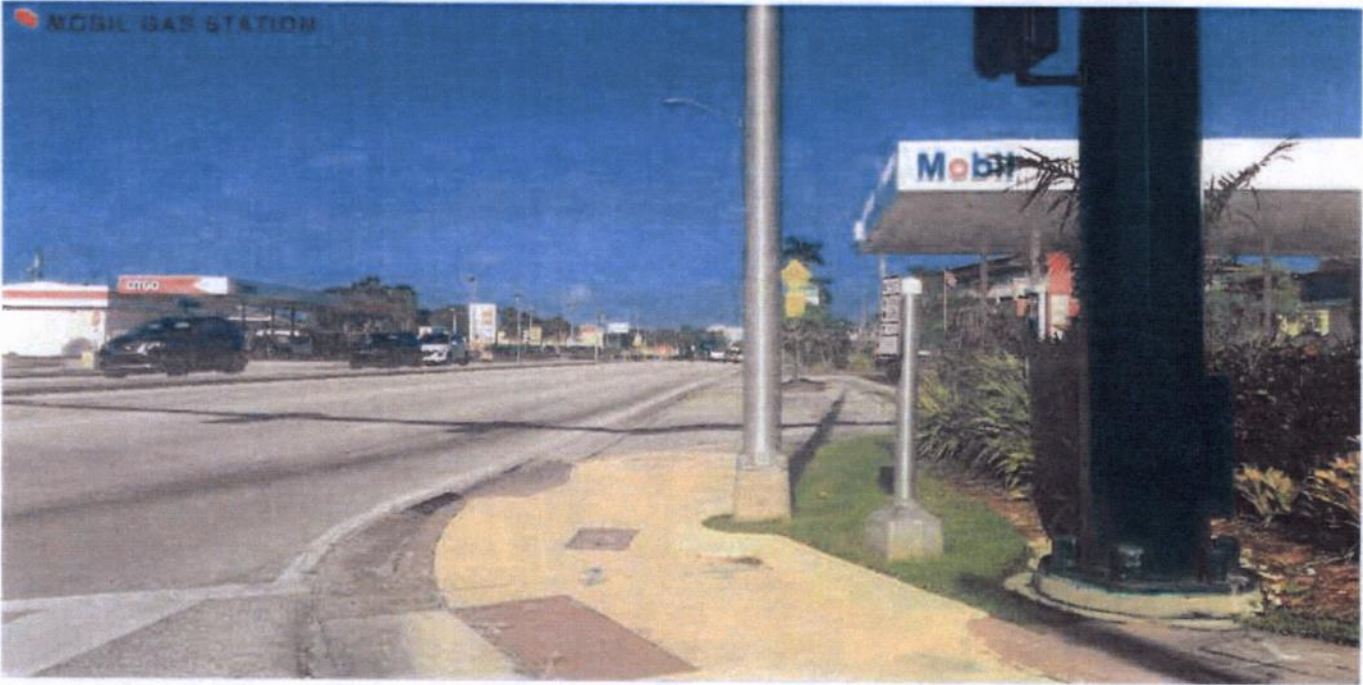
Figure 132 Image of site from Southwest Federal Highway.
