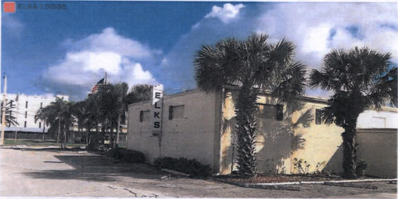
Figure 118 Image of site from South Kanner Highway.
