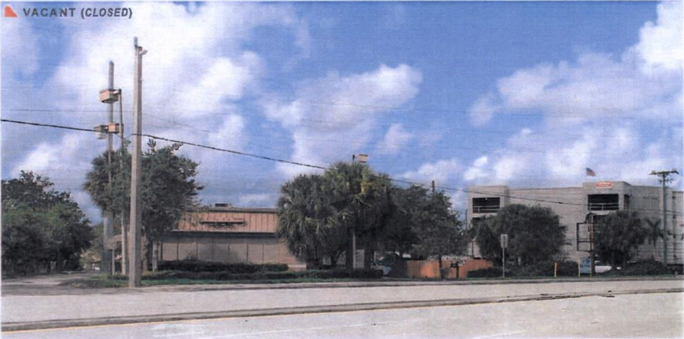
Figure 143 Image of site from Southwest Federal Highway.
