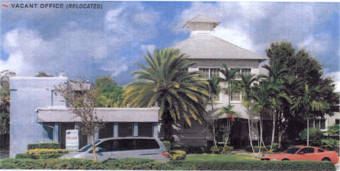
Figure 161 Image of site from Southwest Federal Highway.
