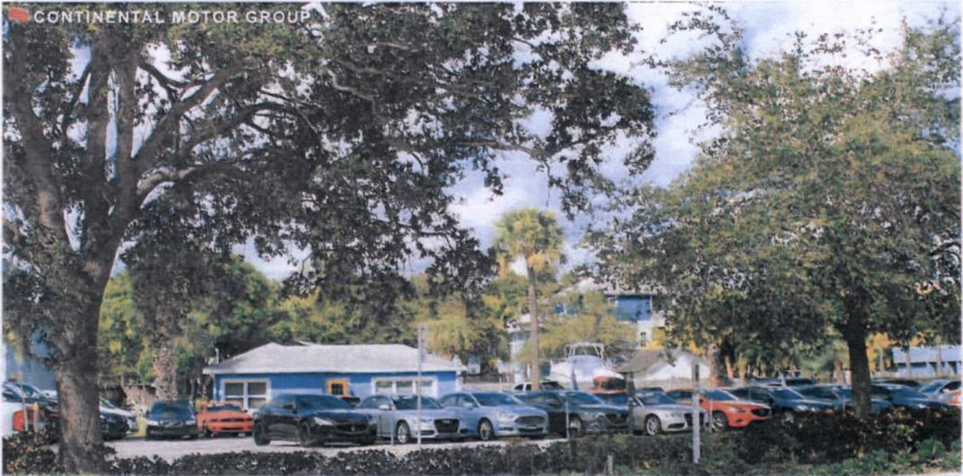
Figure 159 Image of site from Southwest Federal Highway.
