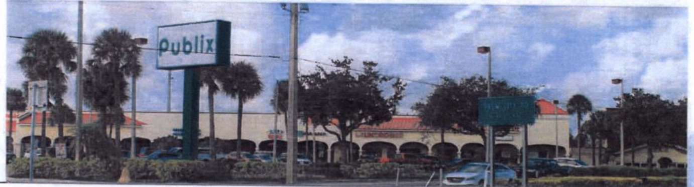
Figure 137 Image of site from Southwest Federal Highway.
