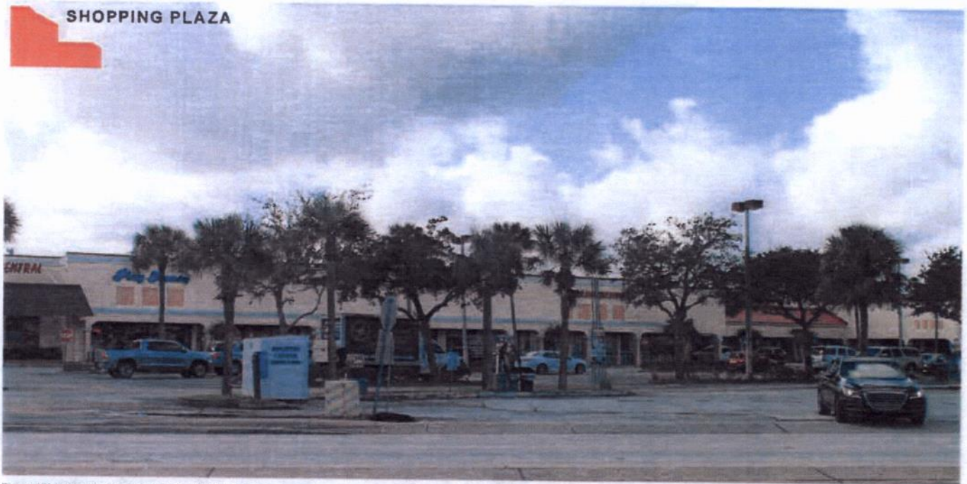
Figure 136 Image of site from Southwest Federal Highway.
