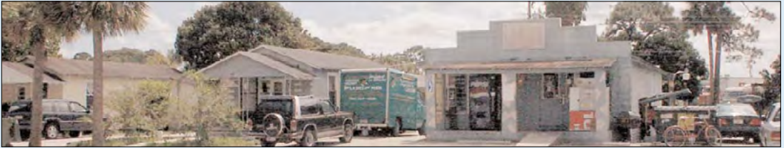
Figure 48 The above image is from 2003 and includes the Taylor Grocery Store. Since that time, these buildings have been demolished.
