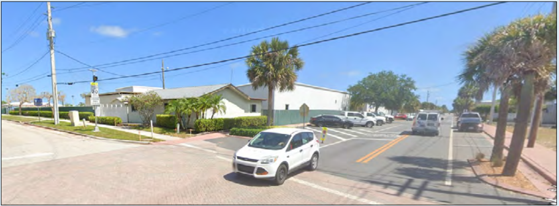
Figure 36 View of the vehicle maintenance facility in 2022.
