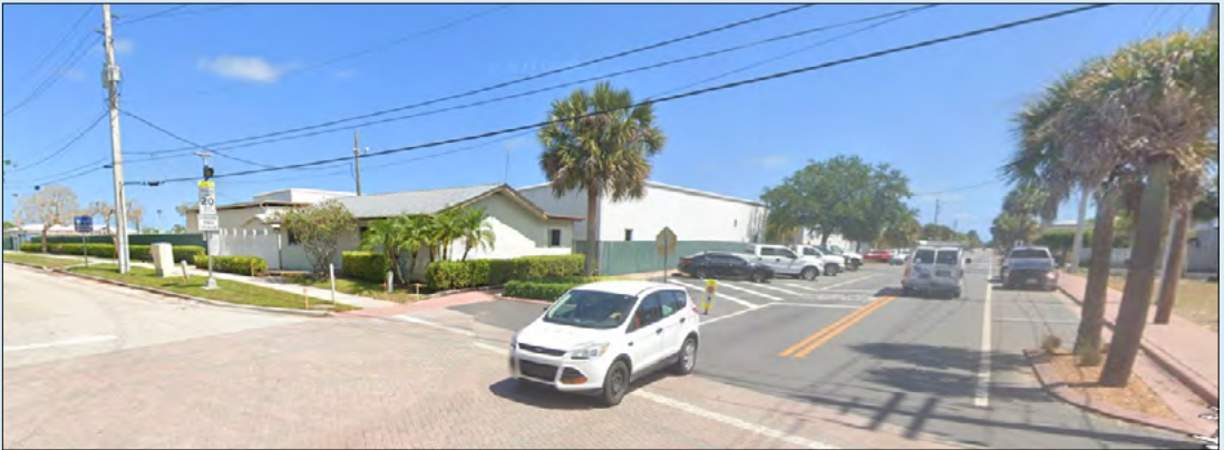
Figure 36 View of the vehicle maintenance facility in 2022.
