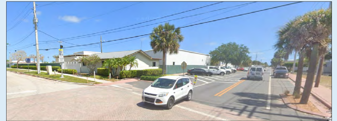
Figure 36 View of the vehicle maintenance facility in 2022.
