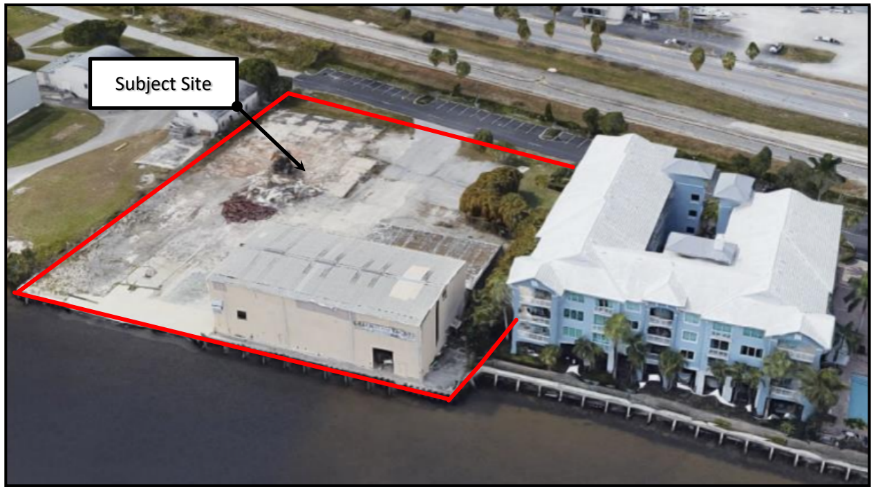
Exhibit 1.1: Historic Site Conditions (Source: Google Earth Aerial)
