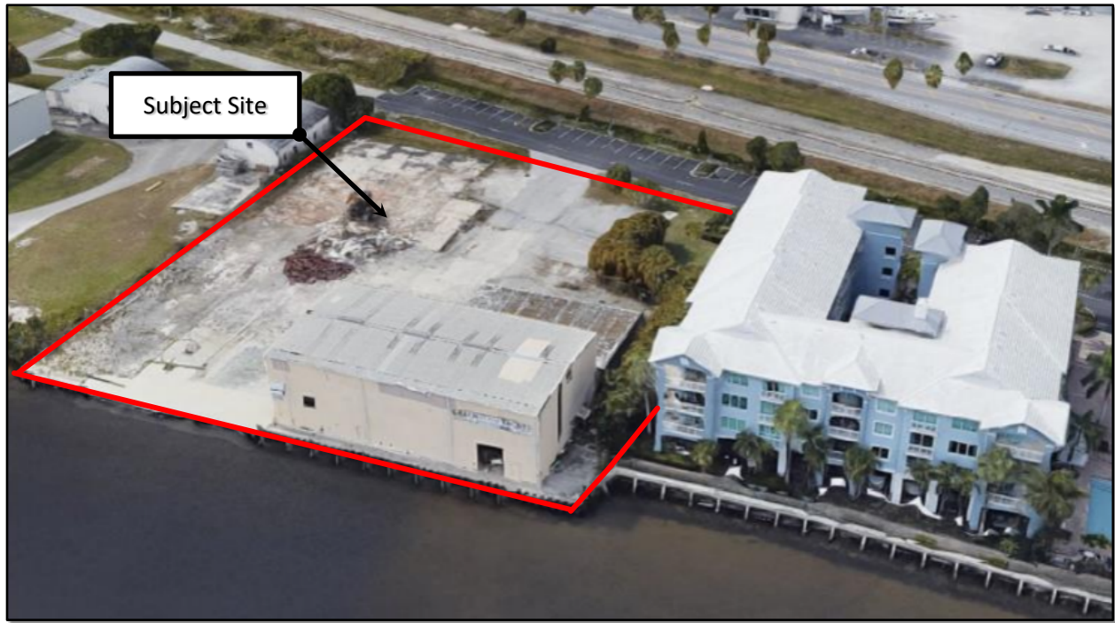
Exhibit 1.2: Historic Site Conditions ( Source: Google Earth Aerial )
