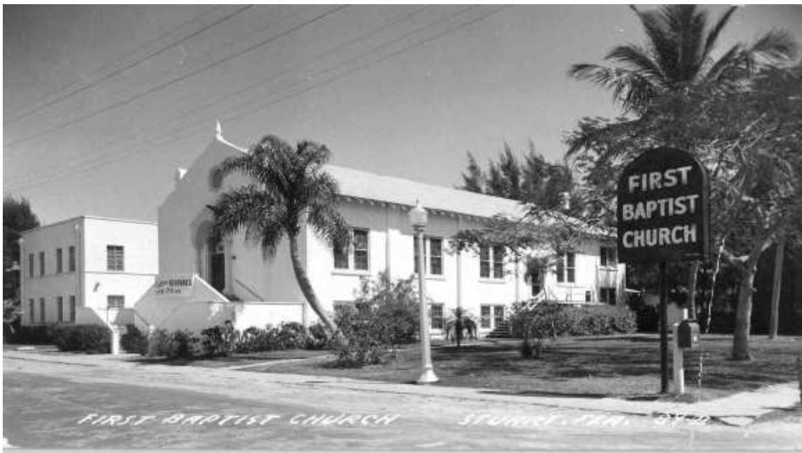
FIGURE 21. FIRST BAPTIST CHURCH, 200 AKRON AVE
