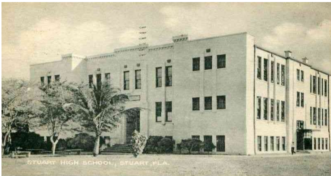
FIGURE 19. STUART HIGH SCHOOL, 500 OCEAN BLVD
