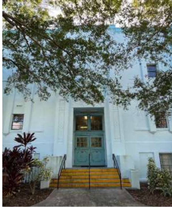
FIGURE 43. STUART HIGH SCHOOL, 500 SW OCEAN BOULEVARD
