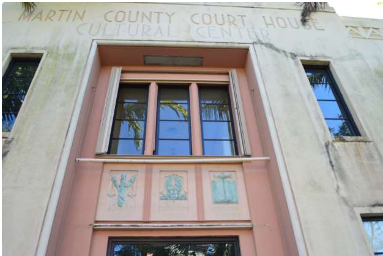
FIGURE 63. ART DECO, MARTIN COUNTY COURTHOUSE, 100 OCEAN BLVD
