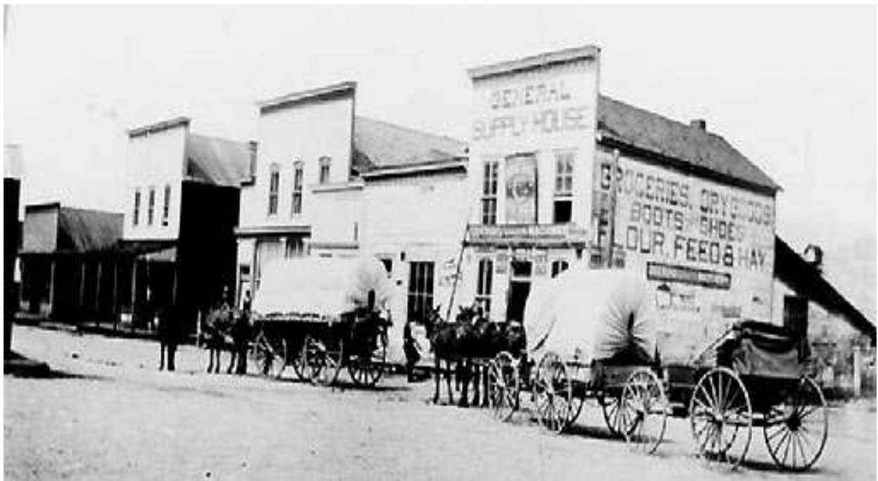
FIGURE 50. FALSE FRONT WOOD FRAME COMMERCIAL BUILDINGS COLORADO
