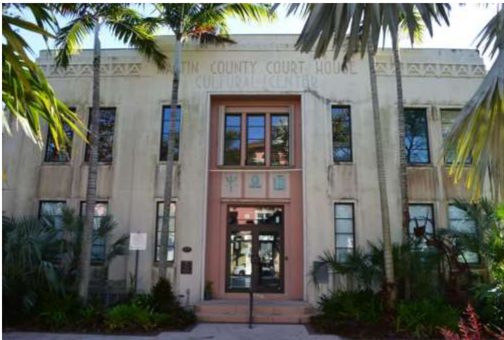
FIGURE.37. MARTIN COUNTY COURTHOUSE, 100 SE OCEAN BOULEVARD
