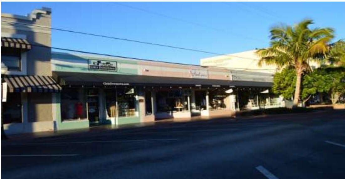
FIGURE 51-52. 27-29 FLAGLER AND PRESSEL BUILDING FLAGLER AVENUE
