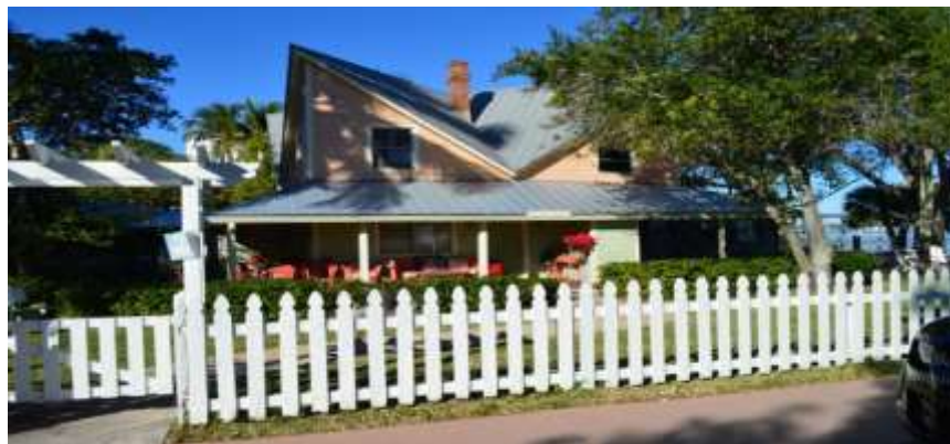
FIGURE 57. THE OWL HOUSE, 100 COLORADO AVENUE
