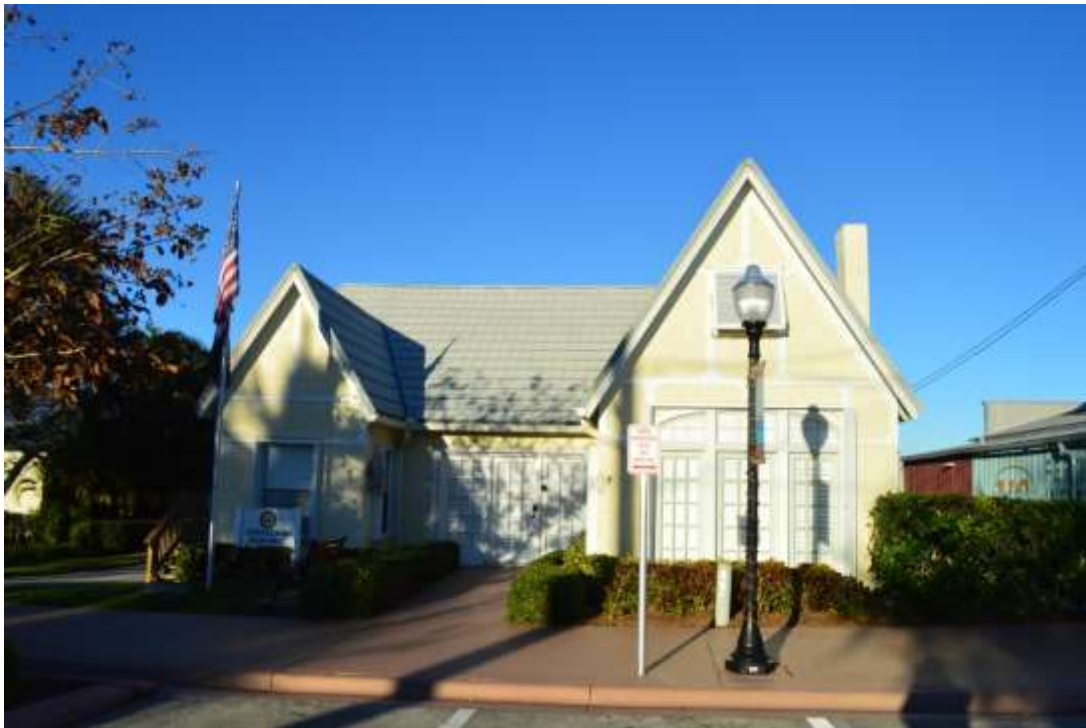
FIGURE 64. TUDOR REVIVAL, CRARY HOUSE, 171 SW FLAGLER AVE
