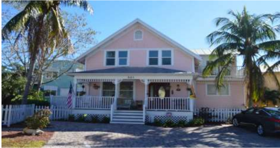
FIGURE 56. SAM MATHEWS HOUSE, 501 AKRON AVENUE
