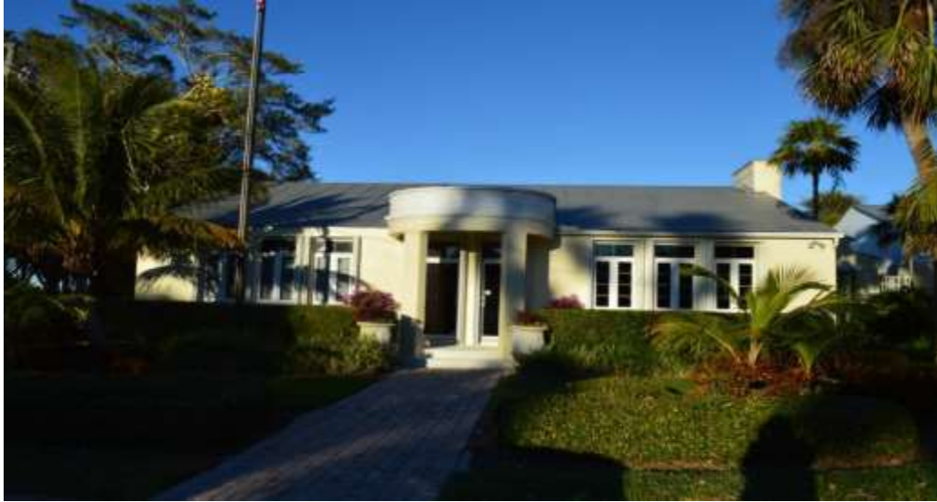
FIGURE 38. FEDERAL RECREATION BUILDING, 201 SW FLAGLER AVENUE
