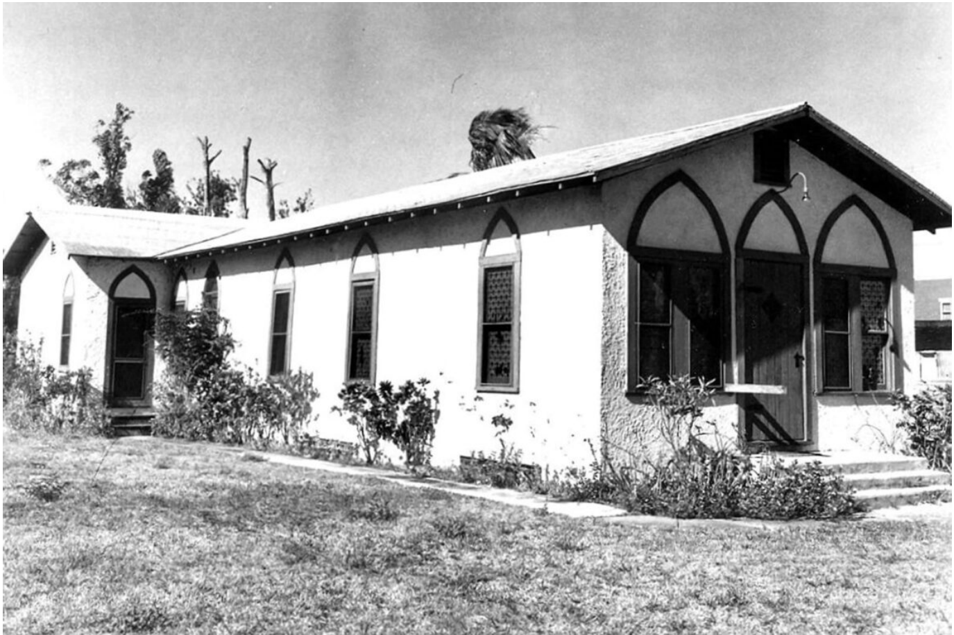
The building that served as the community's first church was purchased by local Episcopalians, moved to West Third Street, and dedicated as St. Mary's Episcopal Church in 1932. (Photo courtesy Leona Rue Luckhardt)
