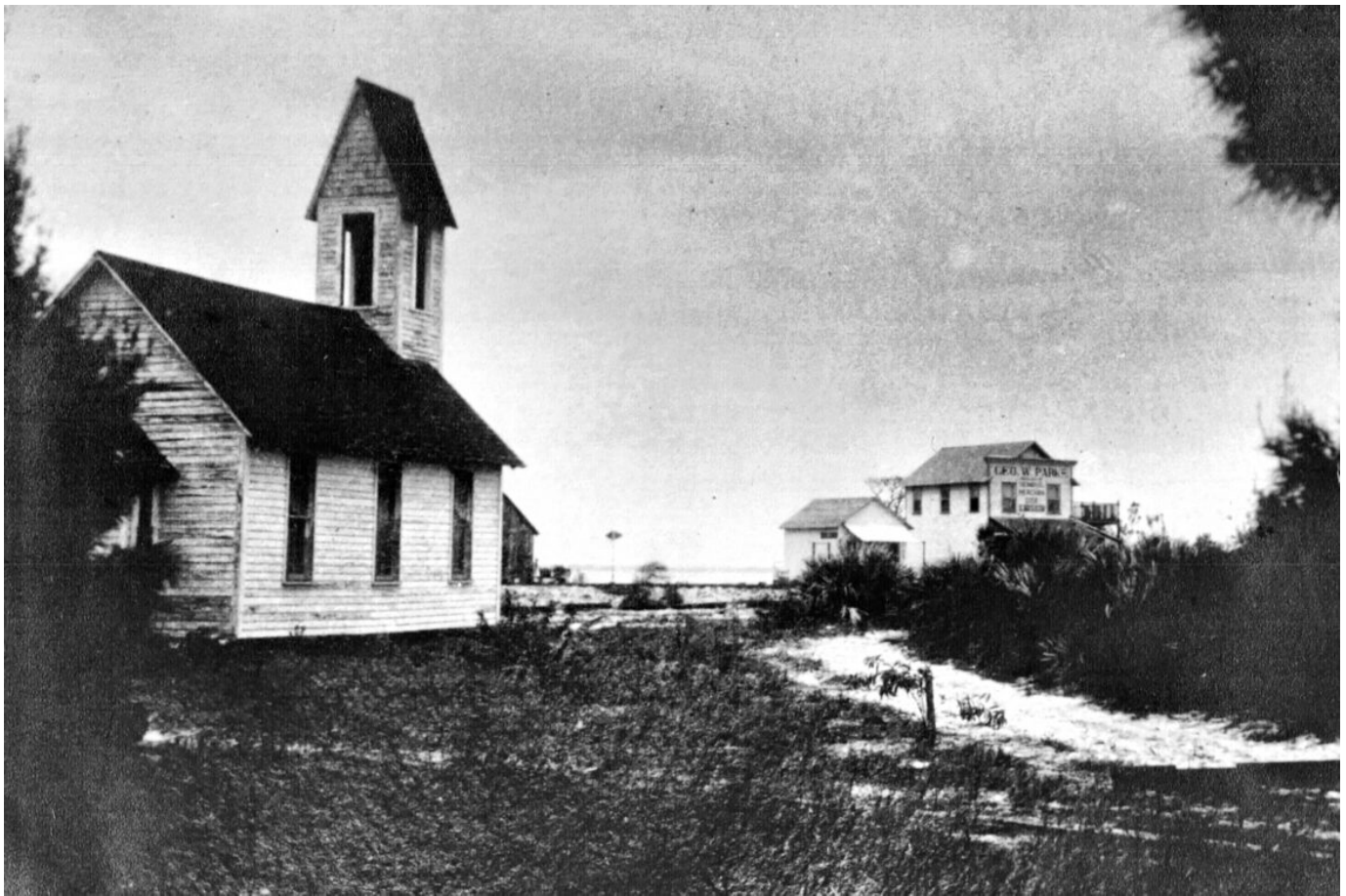
This little Methodist Church, completed shortly before Potsdam's name was changed to Stuart in June 1895, was the community's only house of worship for many years. (1902, Thurlow / Ruhnke Collection)
