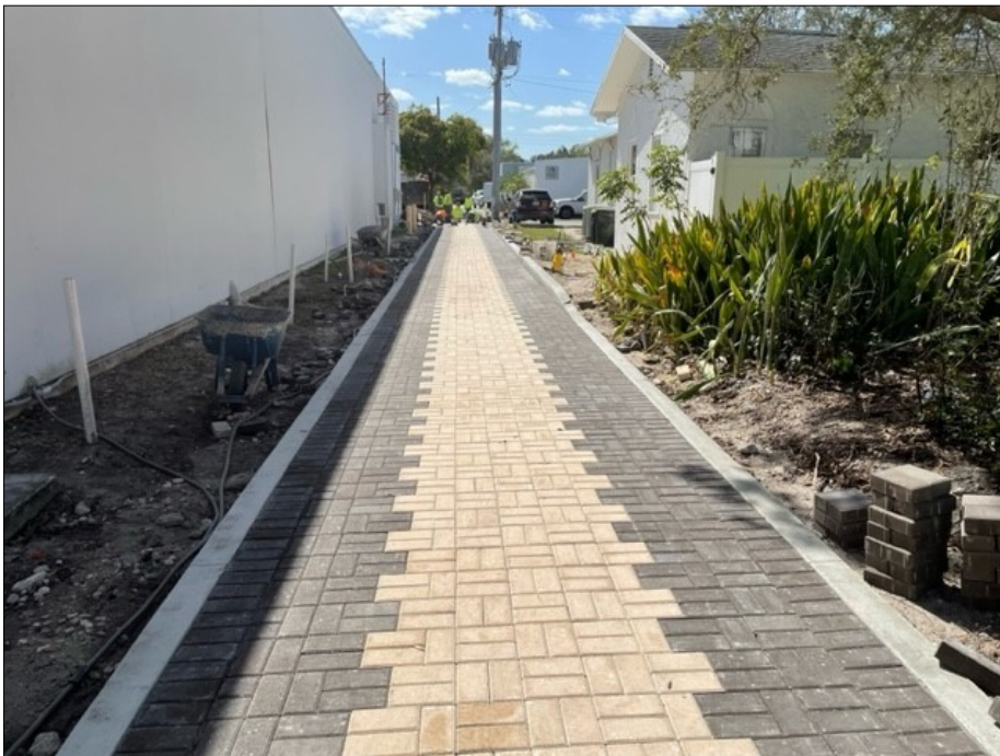
Alleyway Work in Progress
