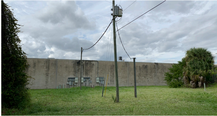
OVERHEAD + UNDERGROUND UTILITIES
