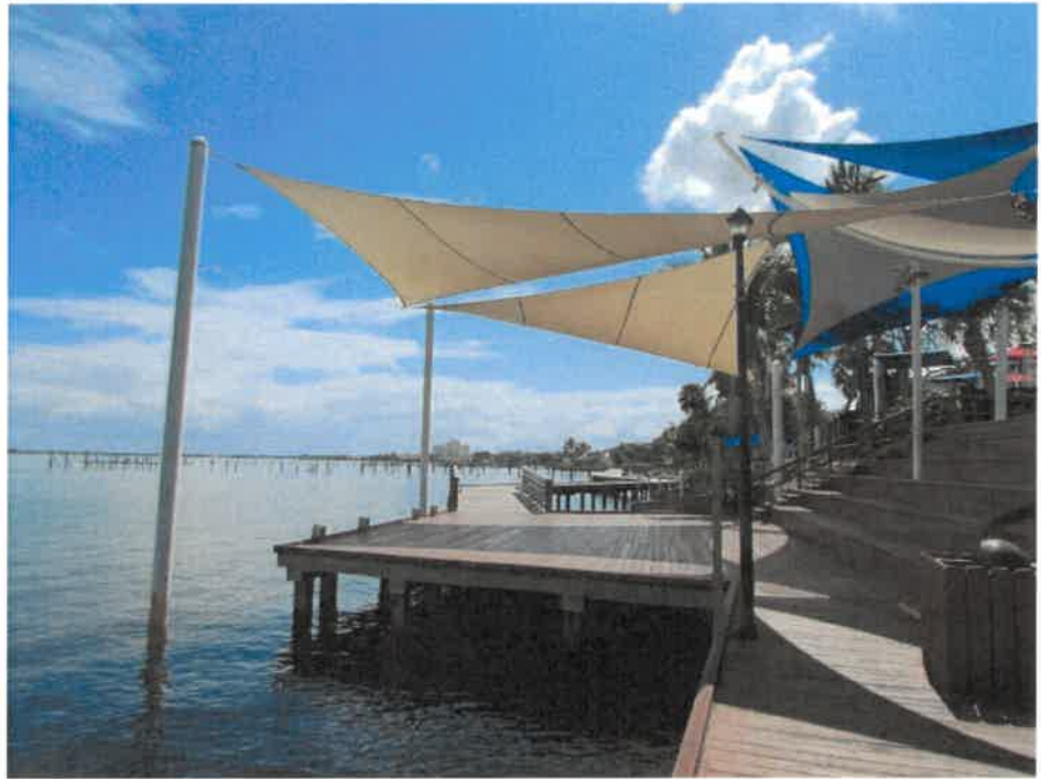
Figure 1: St. Lucie River Boardwalk. Downtown Stuart
