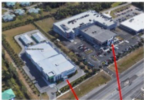
EXTRA SPACE STORAGE (Commercial / 4 story) Martin County Project TOYOTA OF STUART (Commercial / 2 story dealership + 4 story parking structure) Martin County Project
