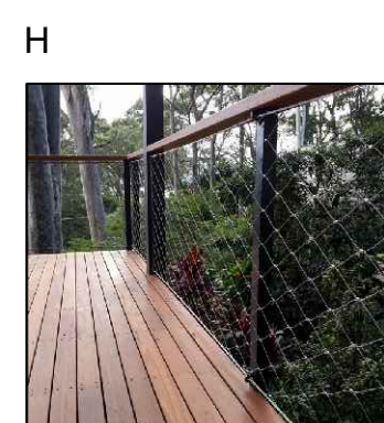
H GUARD RAILS- JACOB ROPE SYSTEMS STAINLESS STEEL WIRE MESH W/ FAUX WOOD TOP-RAIL
