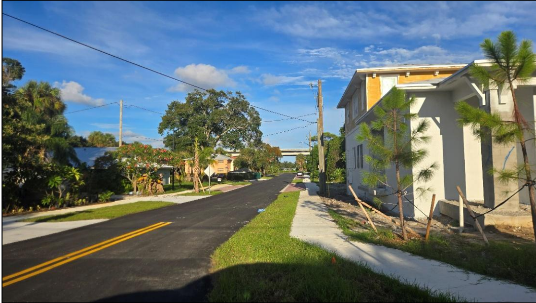
VIEW ALONG NORTH PINE DRIVE
