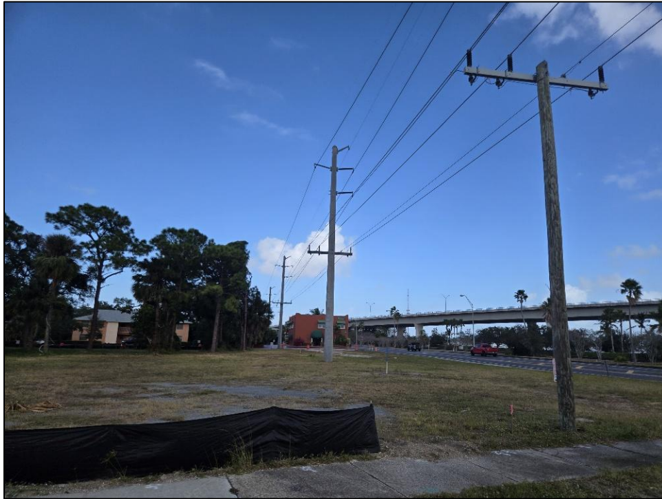
VIEW OF OVERHEAD POWERLINES
