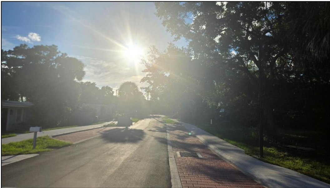
VIEW ALONG NW POINSETTIA STREET
