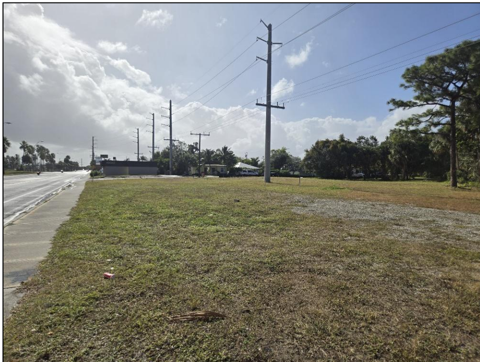
VIEW OF OVERHEAD POWERLINES
