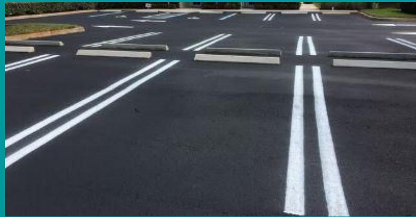
Curb Stops & Restriping
