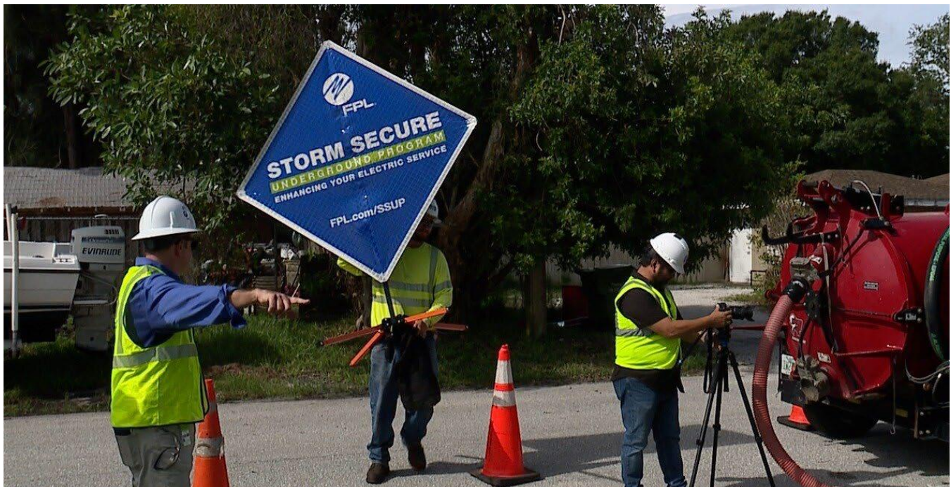
Photo: FPL Installing More Underground Power Lines
