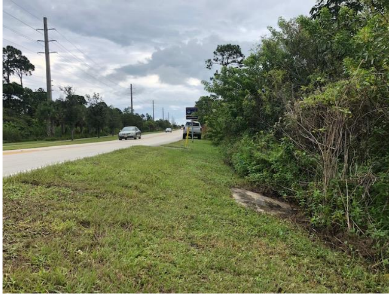
View East along South Side of Baker Road abutting Wetland 1
