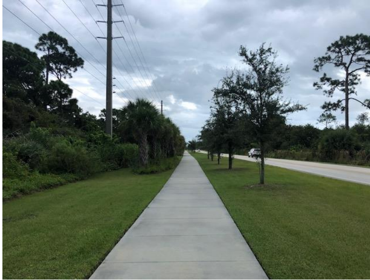
Existing Sidewalk along the north side of Baker Road
