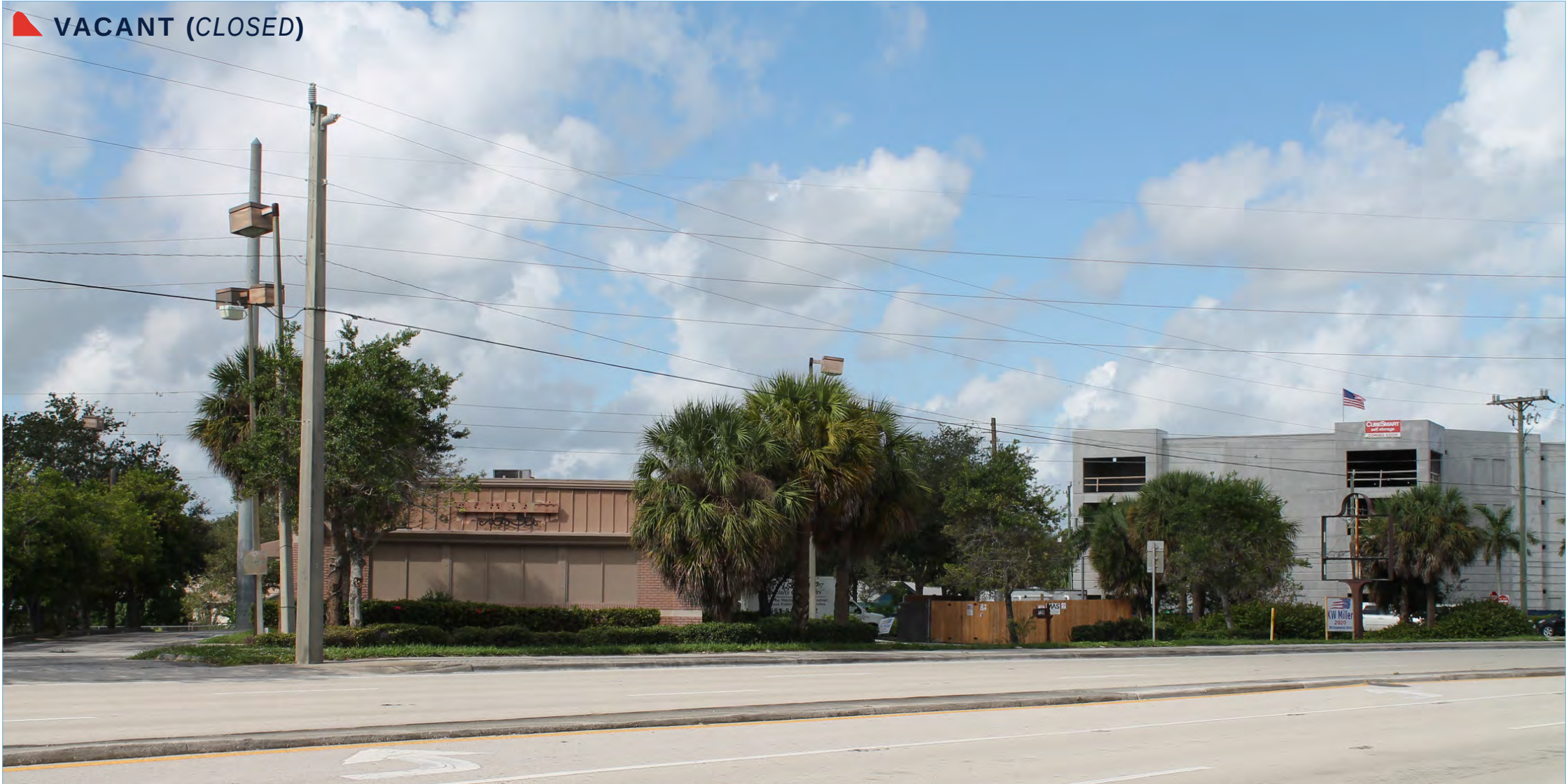
Figure 132 Image of site from Southwest Federal Highway.
