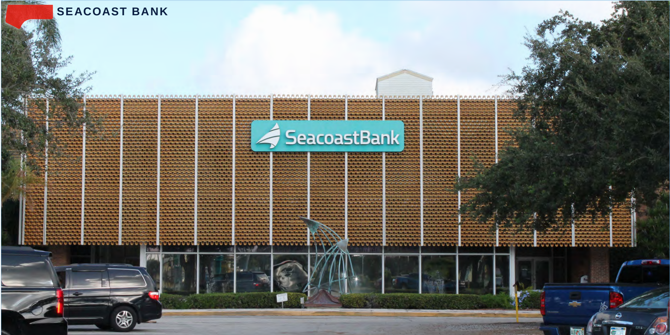
Figure 115 Image of site from Southeast Federal Highway parking lot.
