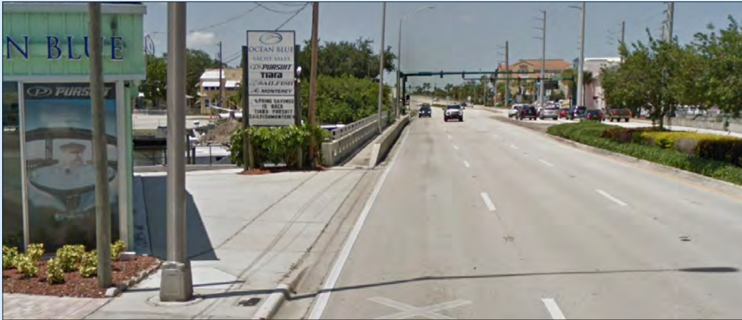
Relocate light poles & remove abandoned driveways.
