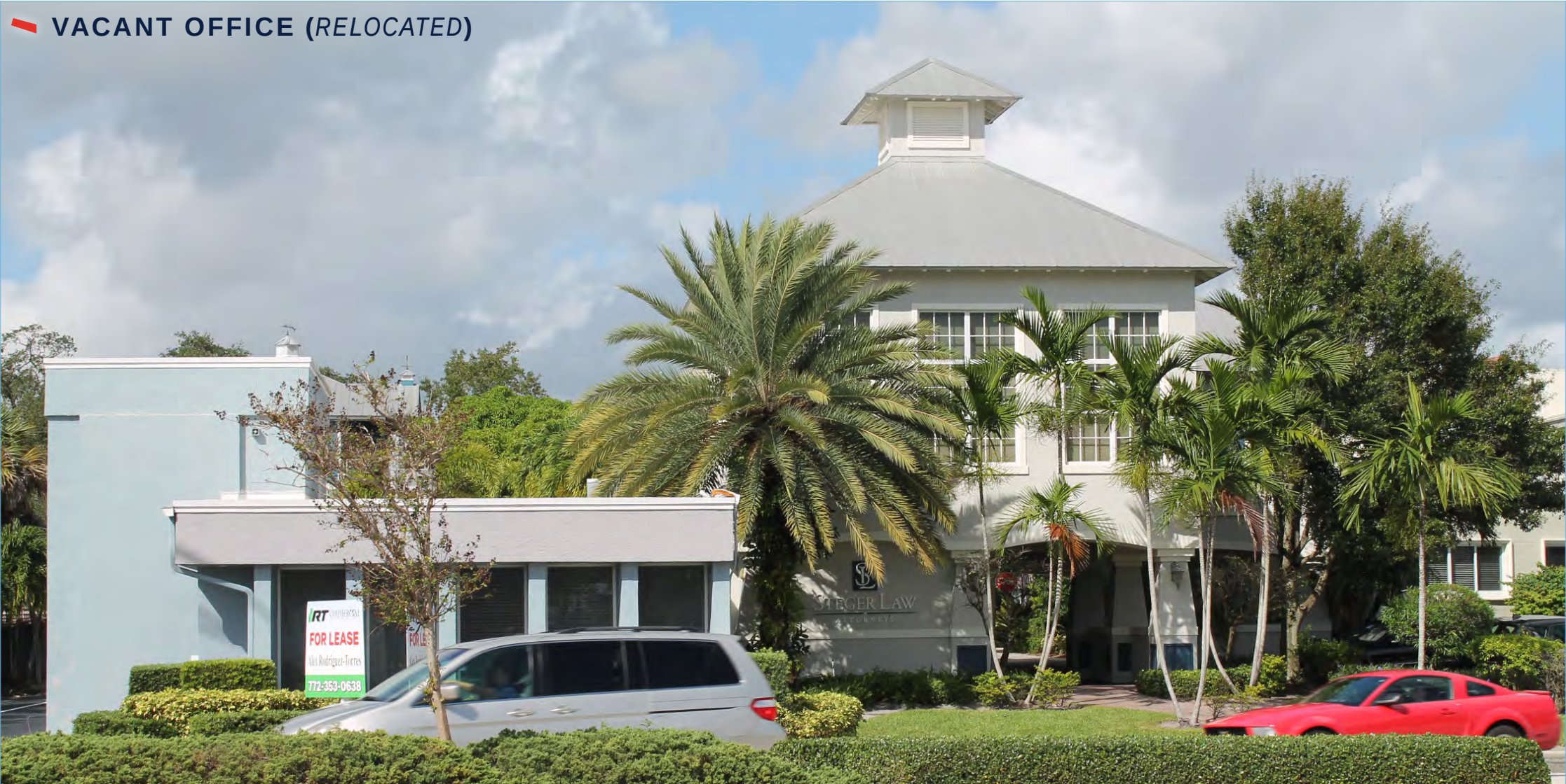
Figure 150 Image of site from Southwest Federal Highway.
