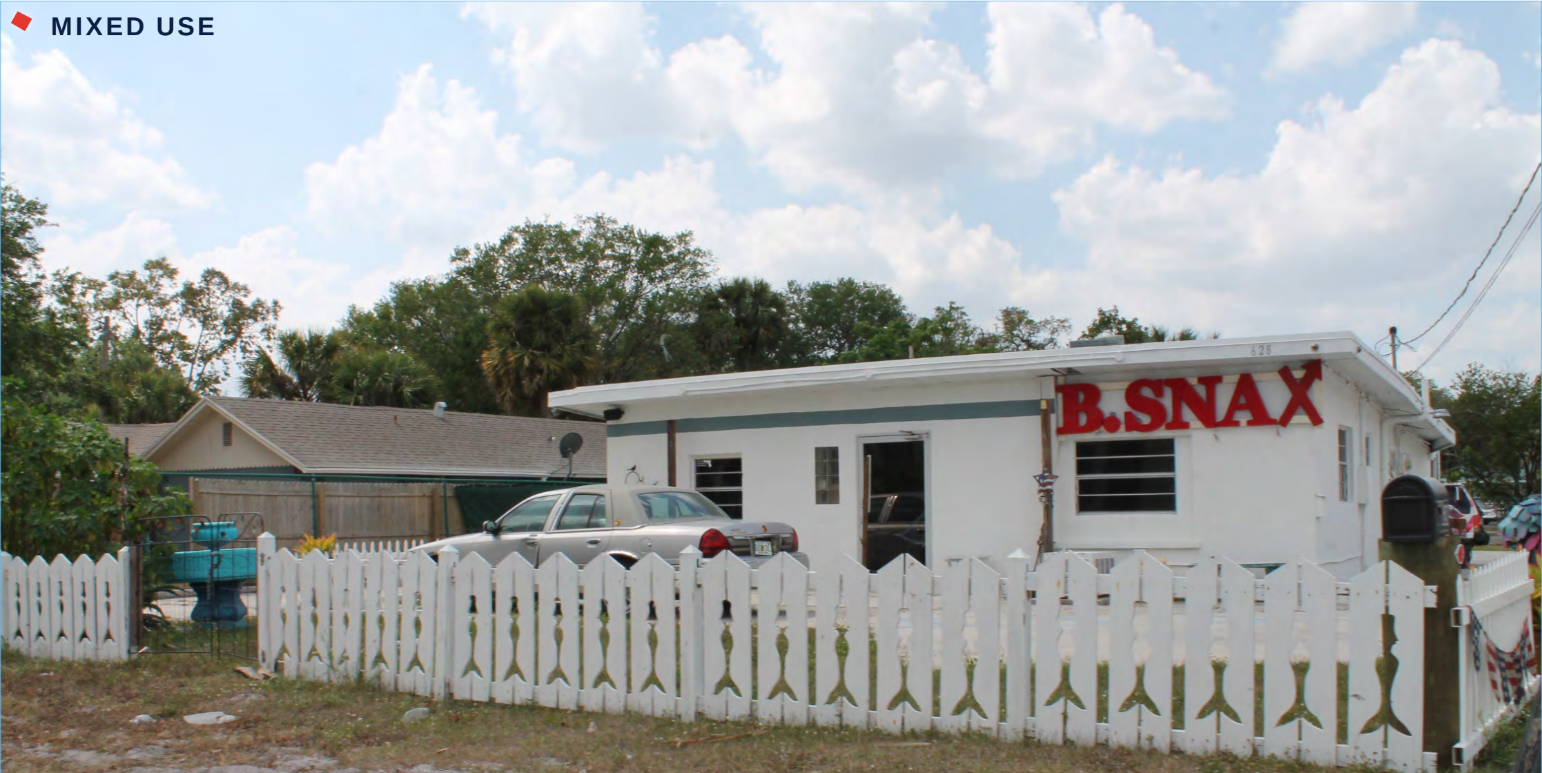
Figure 144 Image of site from Southwest Bryant Avenue.
