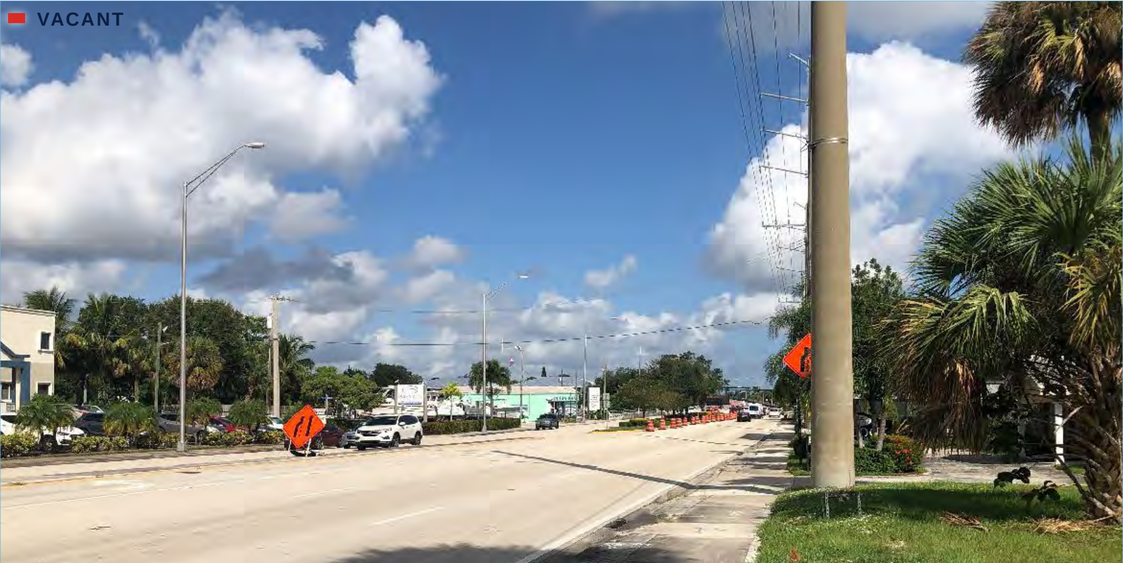
Figure 142 Image of site from Southwest Federal Highway.
