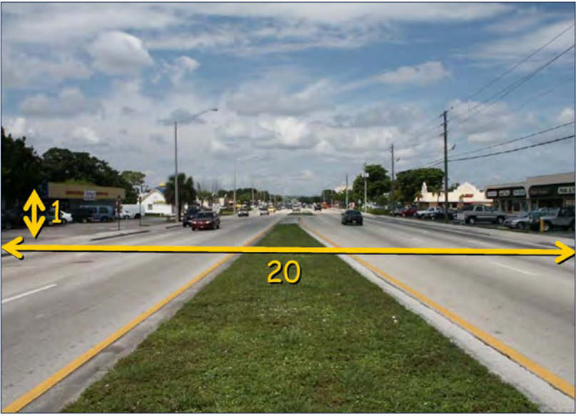
Figure 51 Arterial road with one story buildings set back from the street and parking lots in the front. The public realm has a 1 to 20 ratio.
