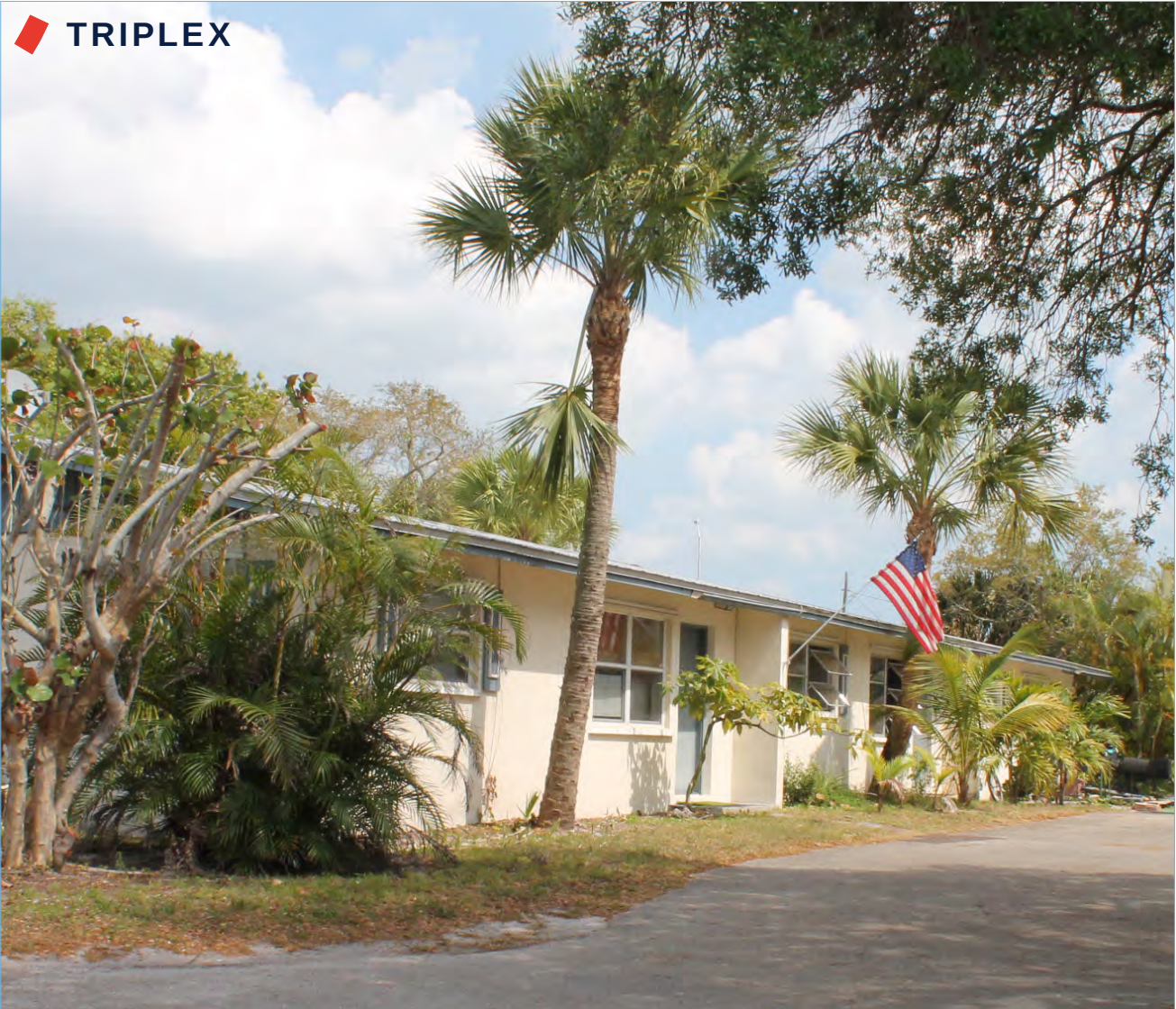
Figure 156 Image of site from Southwest Cleveland Avenue.
