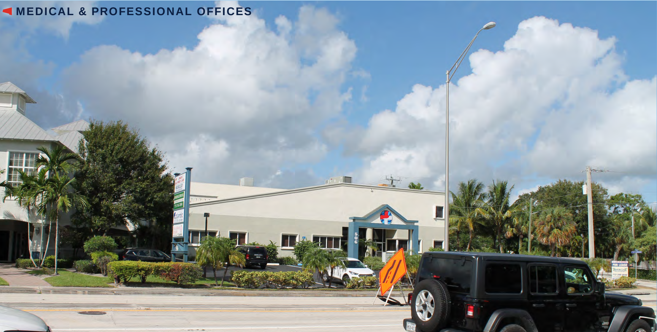
Figure 154 Image of site from Southwest Federal Highway.
