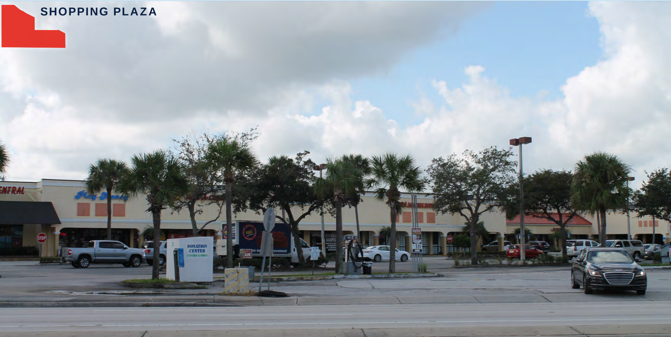
Figure 125 Image of site from Southwest Federal Highway.
