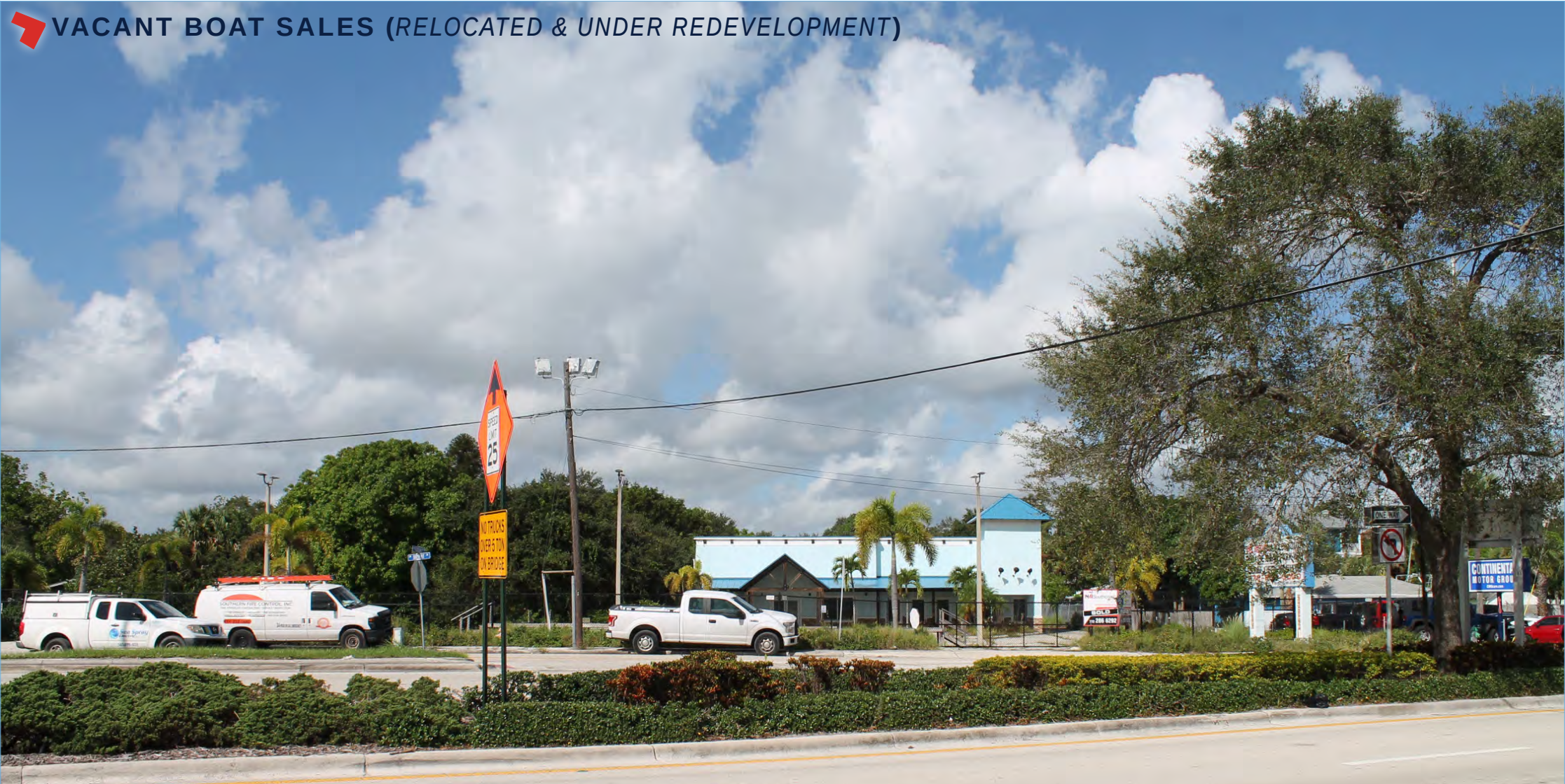
Figure 146 Image of site from Southwest Federal Highway.
