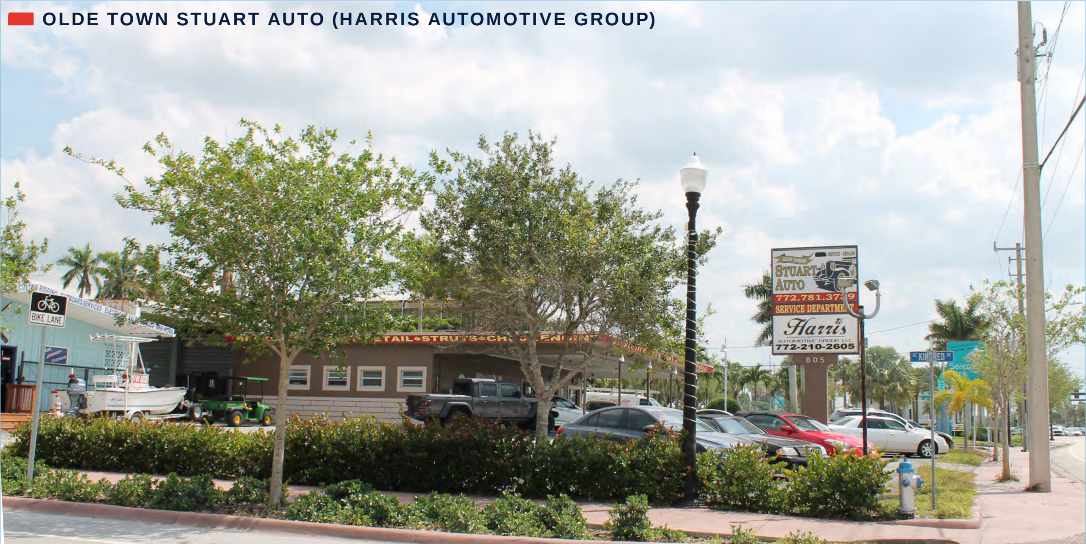
Figure 119 Image of site from South Colorado Avenue.
