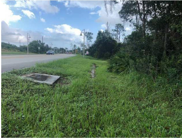
View North along East side of Greenriver Parkway abutting Wetland 1
