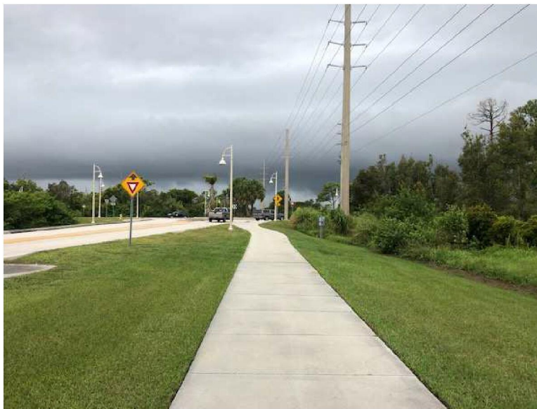
Existing Sidewalk Along the north side of Baker Road
