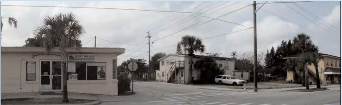
Figure 38 Image above of the existing intersection in 2003.
