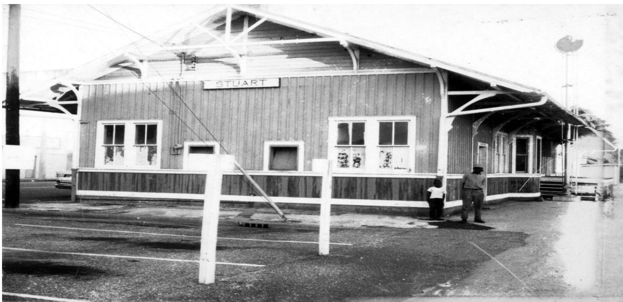
FIGURE 4. SECOND STUART FLORIDA EAST COAST RAILWAY DEPOT, 1913
