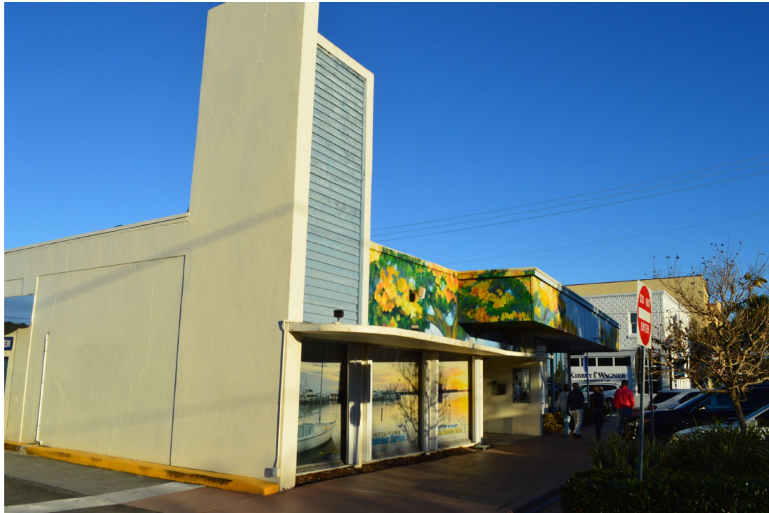
PHOTO 27, Stuart Department Store, 101 SW Flagler Avenue, facing south
