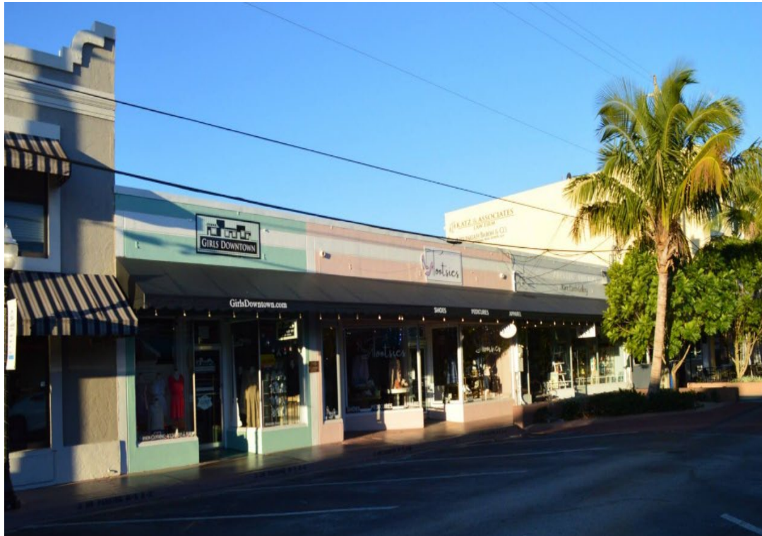
PHOTO 21, Pressel Building, 37-47 SW Flagler Avenue, east side facing west
