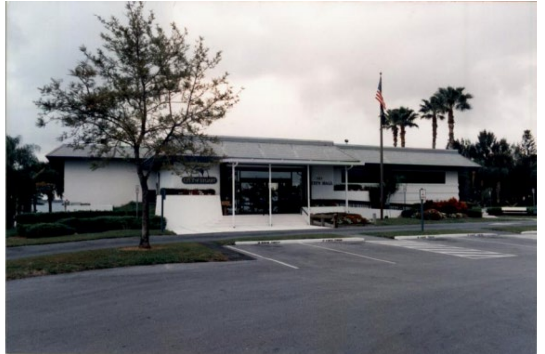
PHOTO 14 Stuart City Hall, 121 SW Flagler Ave. facing east
