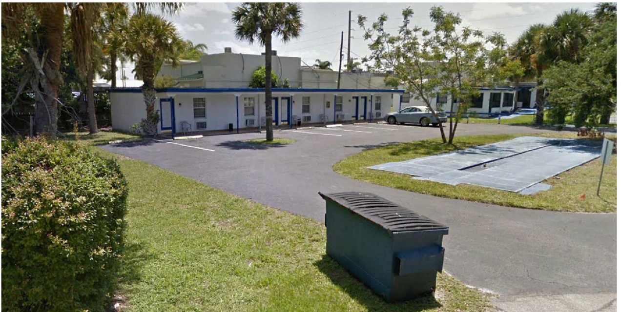
VIEW FROM SW 6 th STREET
