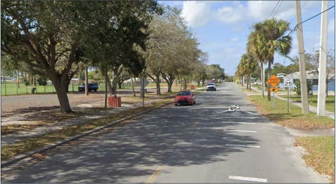
Figure 16 The above image of the street shows the mature trees which provide significant shade.
