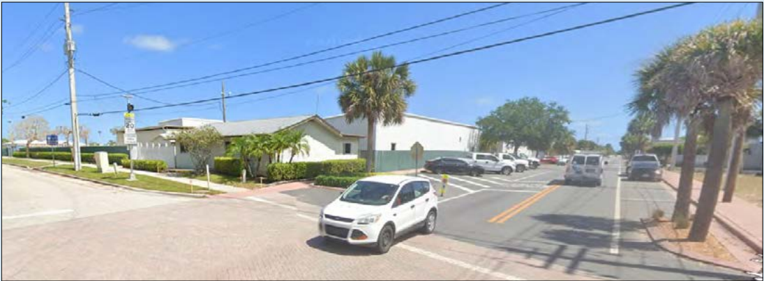
Figure 36 View of the vehicle maintenance facility in 2022.
