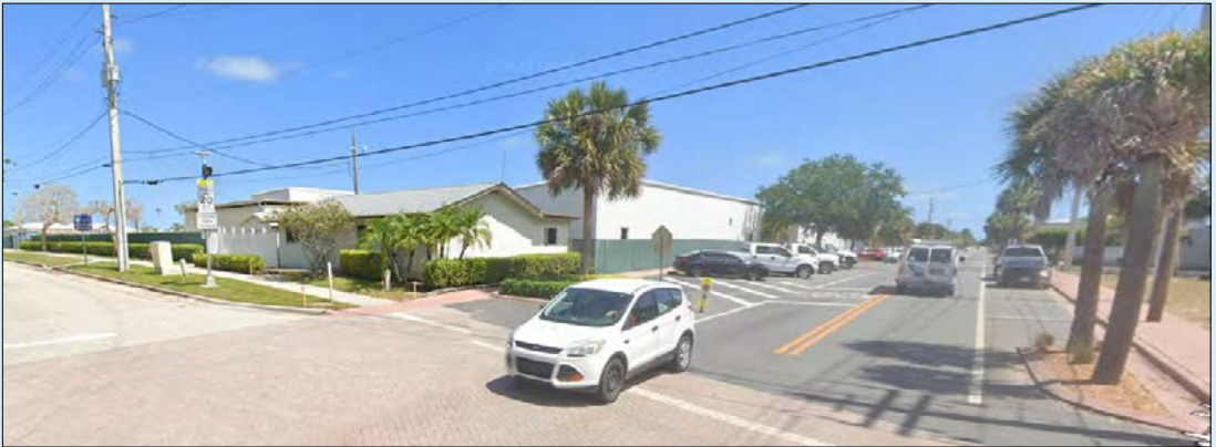
Figure 36 View of the vehicle maintenance facility in 2022.
