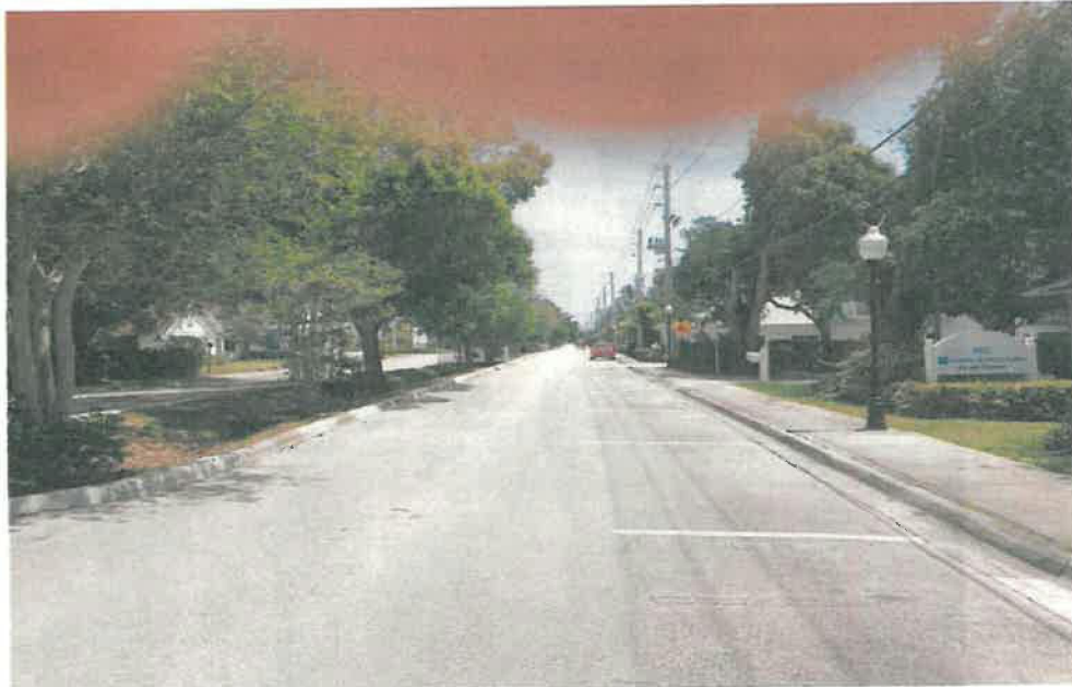
SE Osceola Street looking east.
