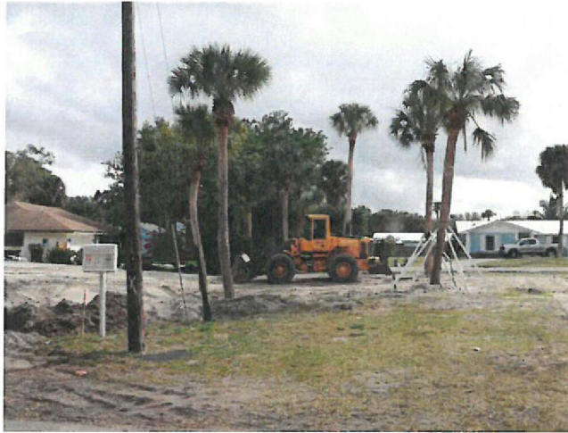
Subject – unopened street right of way
