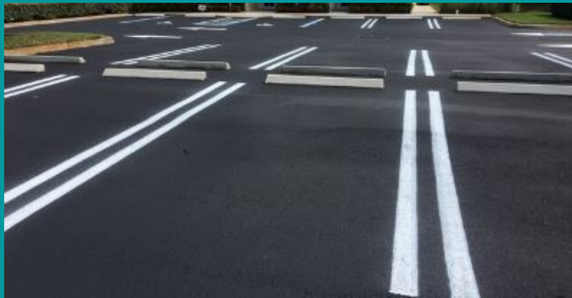
Curb Stops & Restriping
