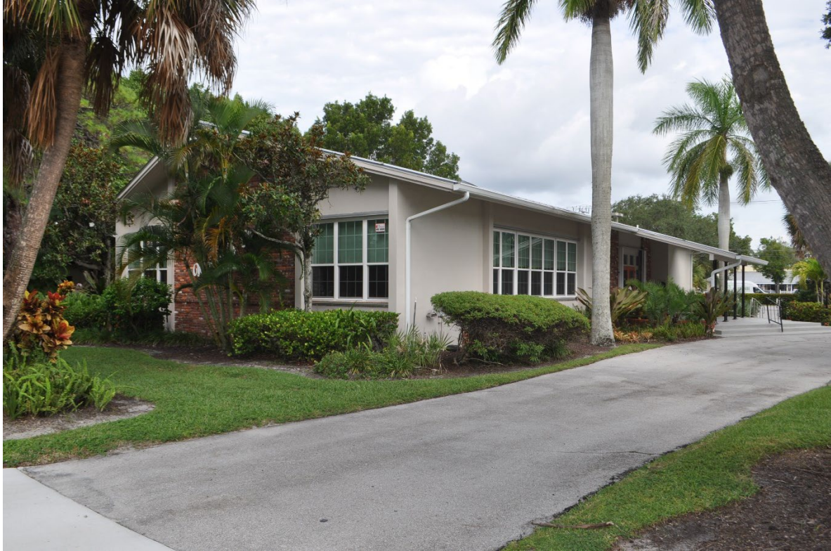
South and east elevations containing PGT impact vinyl 9-over-6 single-hung new windows (above). South elevation containing flying gable over original brick section with lettering and new windows.
