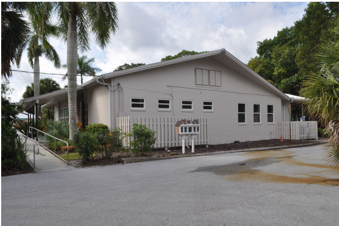
North elevation overlooking parking area. Original flying gable and attic vent louvers. New windows. Flying gable extends out about 60" at the peak. 3 large windows are in the Boardroom.
