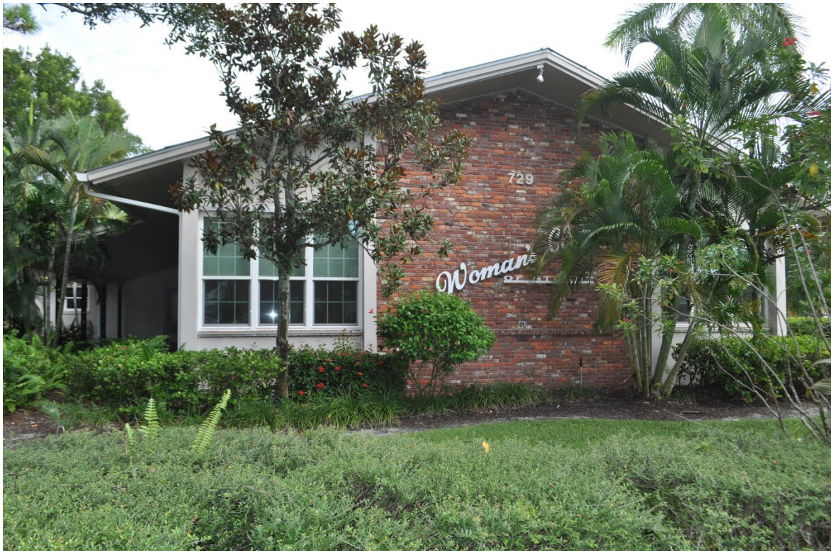
South and east elevations containing PGT impact vinyl 9-over-6 single-hung new windows (above). South elevation containing flying gable over original brick section with lettering and new windows.
