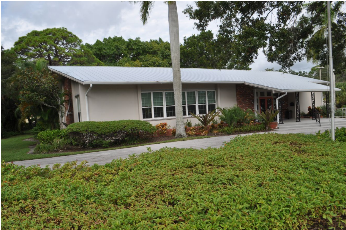
Modifications: standing seam metal roof, impact PGT vinyl windows, French doors.
