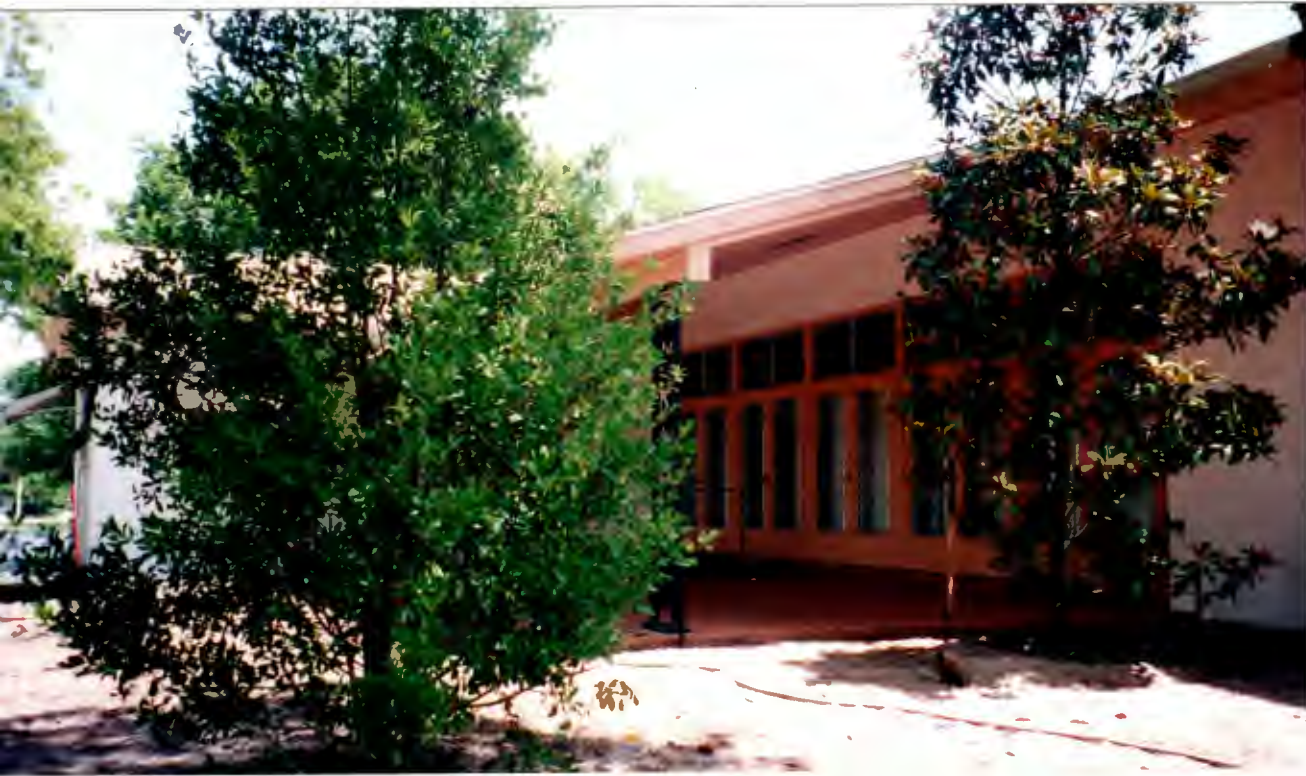
Original jalousie French doors and jalousie transom windows
