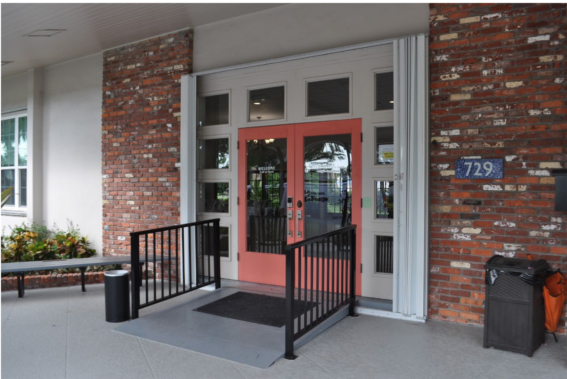
East elevation original and existing wrought iron ivy-design columns (above). Modification: French entry doors and multi-lite panels, removable ADA ramp.
