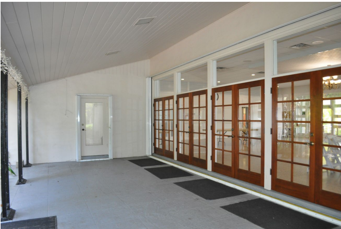
Back patio view towards south. 5 double French doors on left with transoms. Garden on right (above). Back patio view toward north, kitchen door. 5 ½" tongue-and-groove original ceiling. New doors (below).
