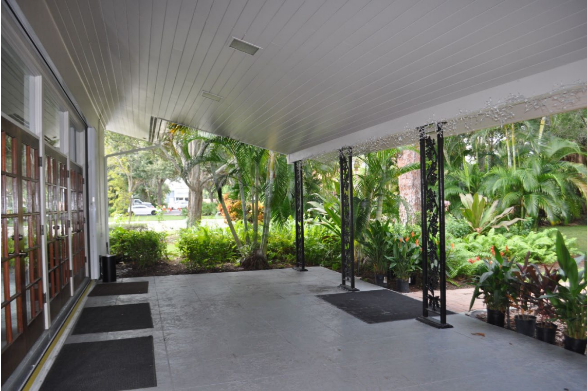
Back patio view towards south. 5 double French doors on left with transoms. Garden on right (above). Back patio view toward north, kitchen door. 5 ½" tongue-and-groove original ceiling. New doors (below).
