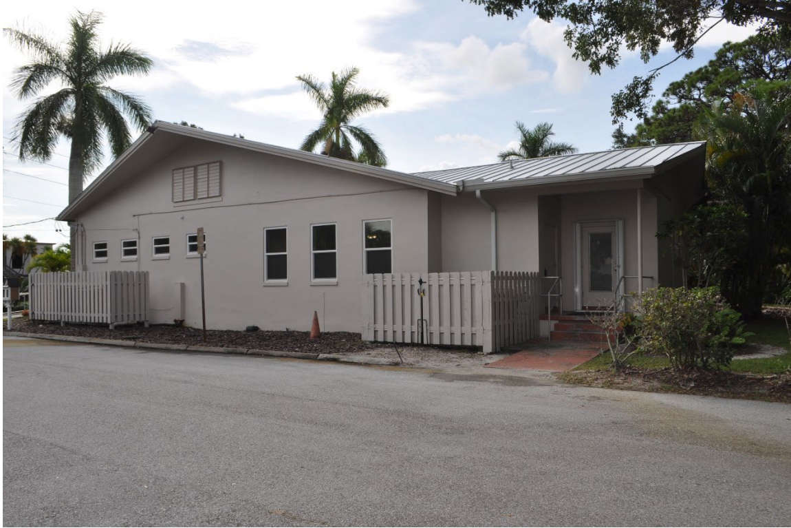
North elevation overlooking parking area. Original flying gable and attic vent louvers. New windows. Flying gable extends out about 60" at the peak. 3 large windows are in the Boardroom.
