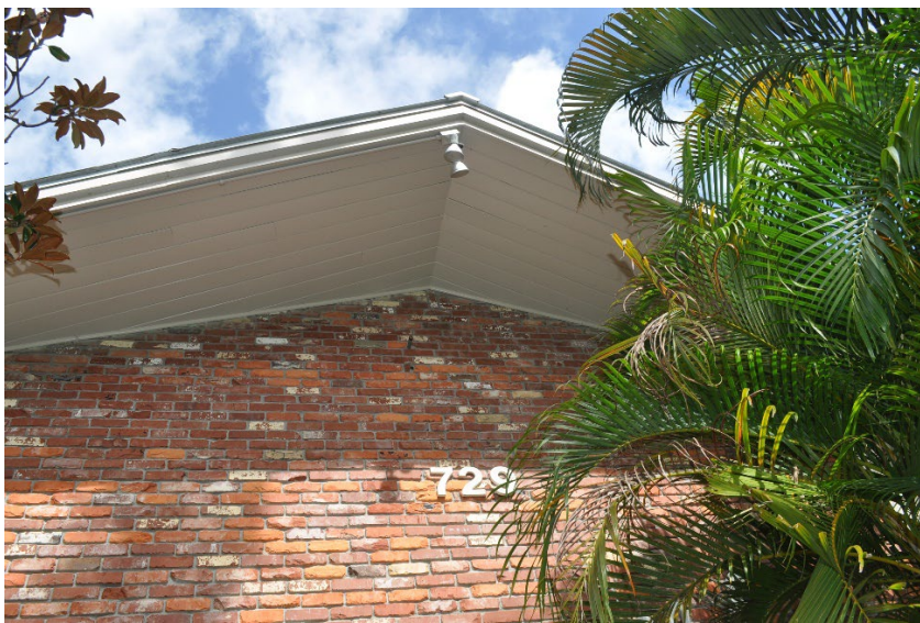
South elevation flying gable.
