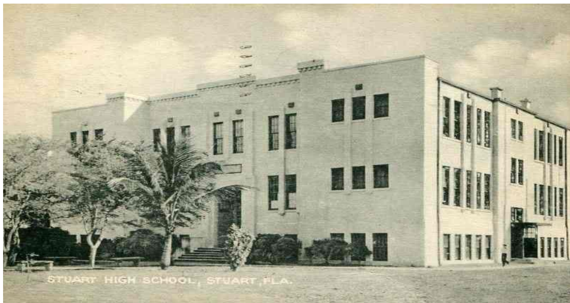
FIGURE 19. STUART HIGH SCHOOL, 500 SE OCEAN BLVD
