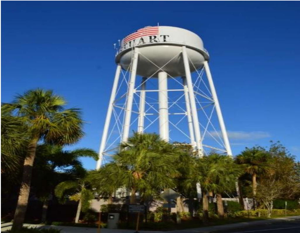
FIGURE 43. CITY OF STUART WATER TOWER, 1959, VICINITY COURTHOUSE
