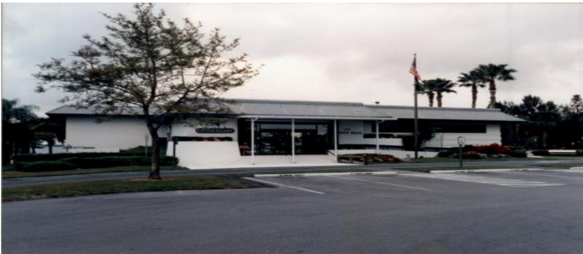
FIGURE 40. 1974 STUART CITY HALL, 121 SW FLAGLER AVENUE
