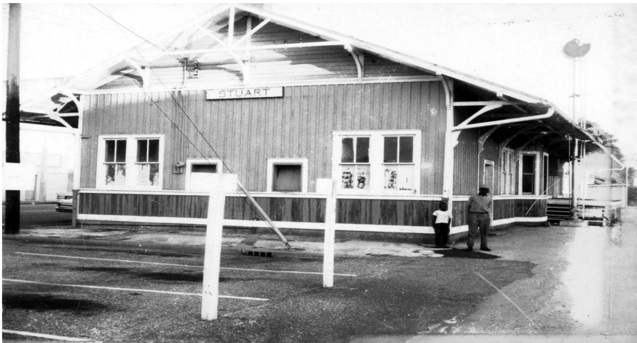
FIGURE 6. SECOND STUART FLORIDA EAST COAST RAILWAY DEPOT, 1913
