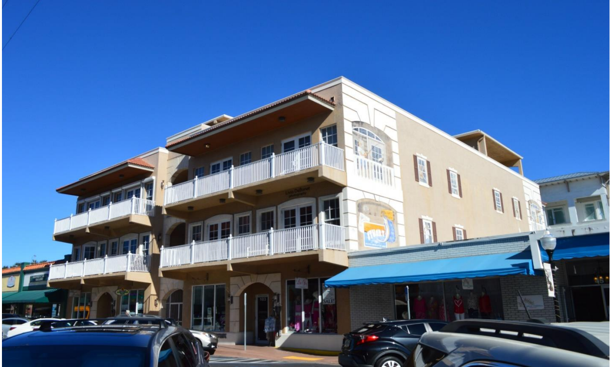
FIGURE 66. MODERN CONDOMINIUMS 47 OSCEOLA STREET DOWNTOWN STUART
