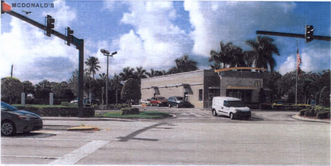
Figure 108 Image of site from Southeast Federal Highway.
