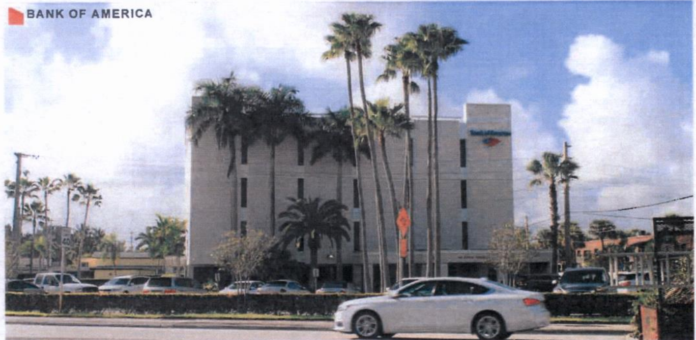
Figure 114 Image of site from Southeast Federal Highway.
