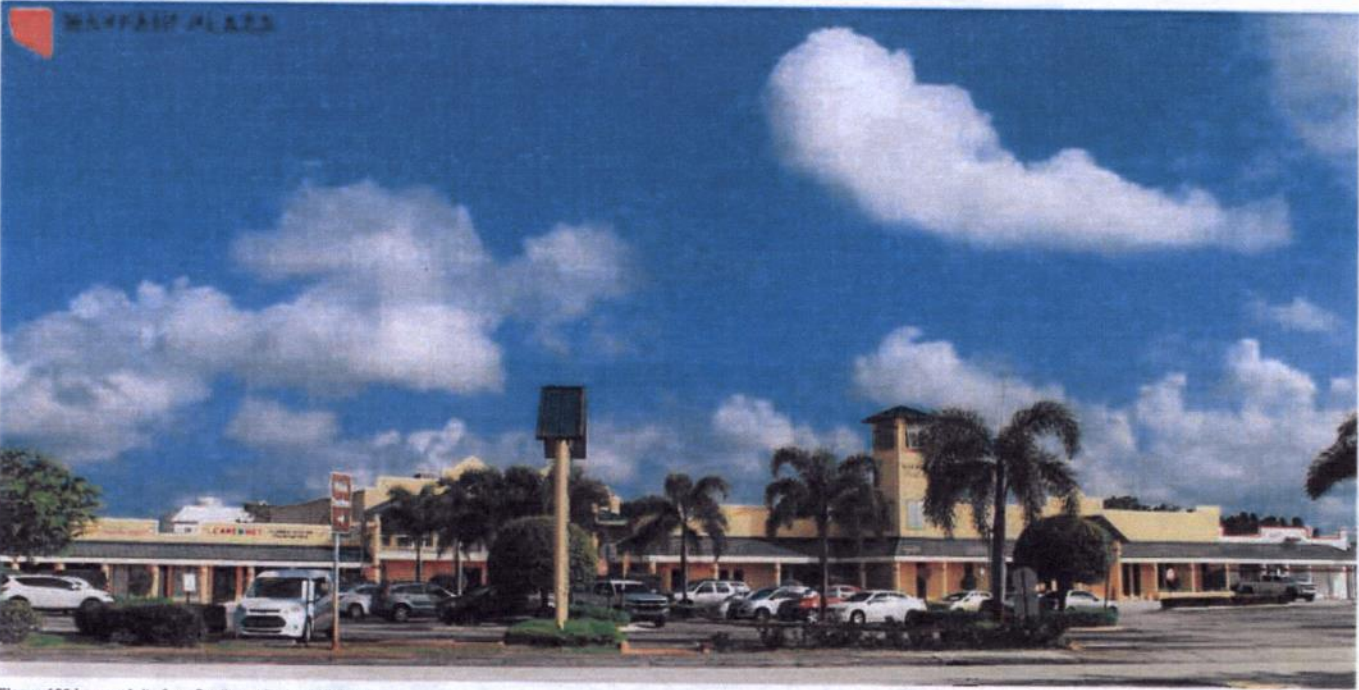
Figure 120 Image of site from Southeast Federal Highway.
