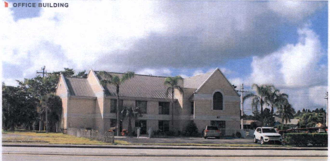
Figure 86 Image of site from Southeast Federal Highway.
