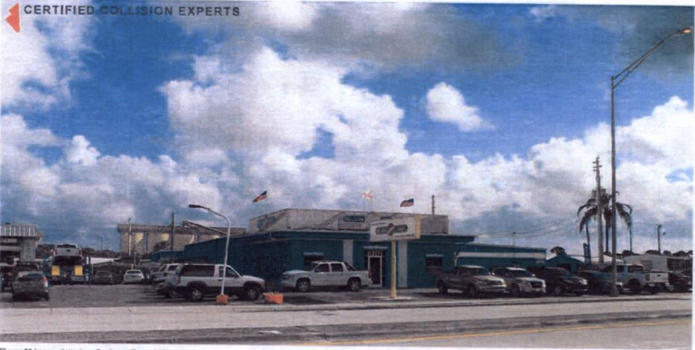
Figure 88 Image of site from Southeast Federal Highway.
