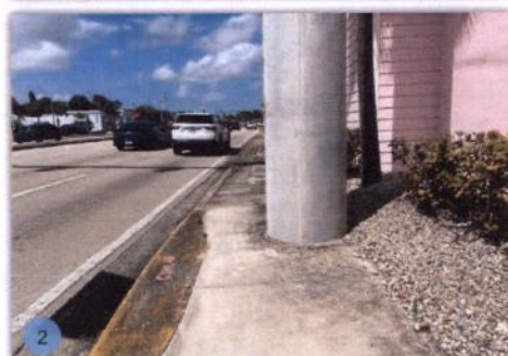
Figure 12 Photo of existing sidewalk condition within the study area at US-1/Federal Highway where a utility pole reduces the clear path significantly.
