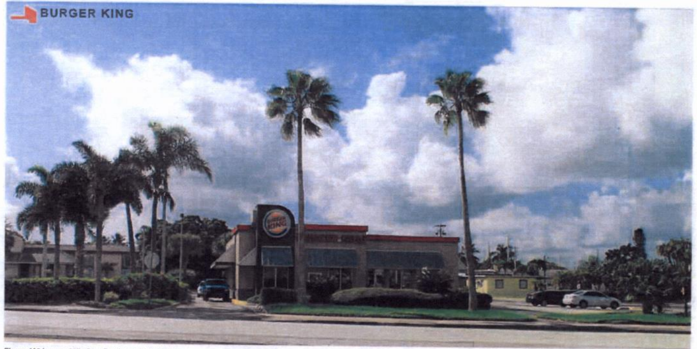
Figure 112 Image of site from Southeast Federal Highway.
