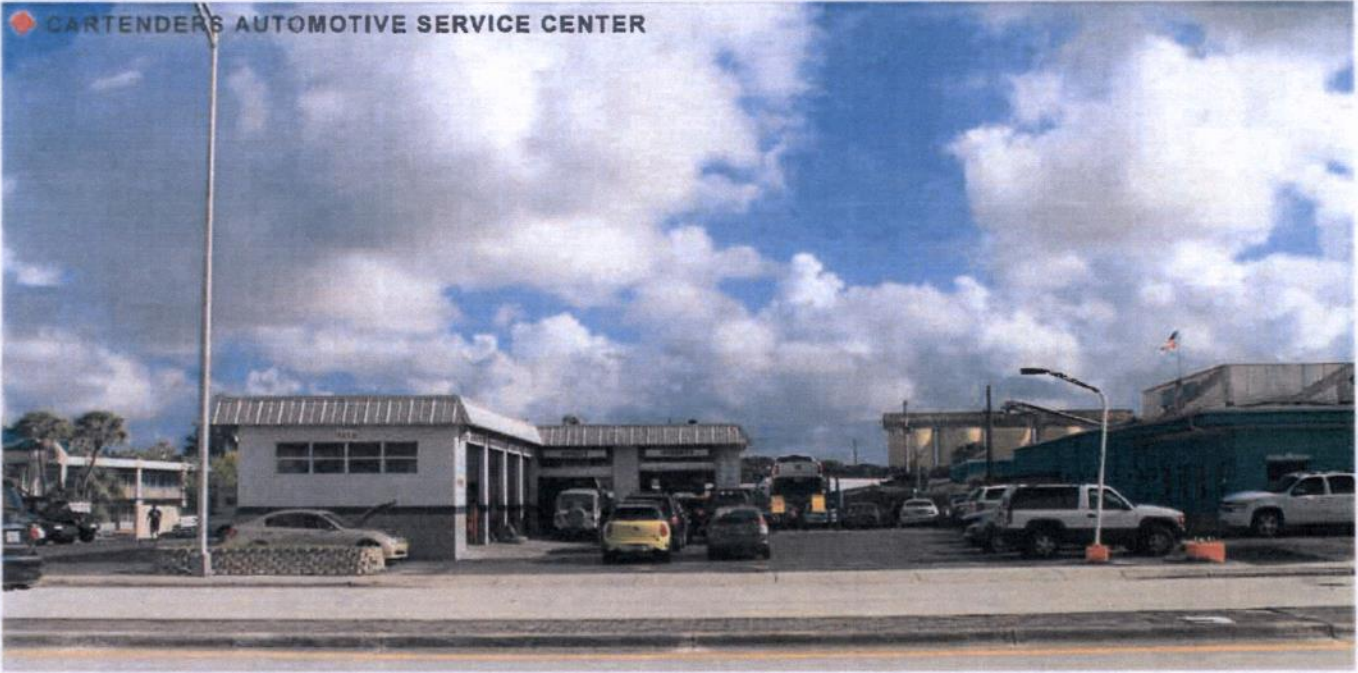
Figure 90 Image of site from Southeast Federal Highway.
