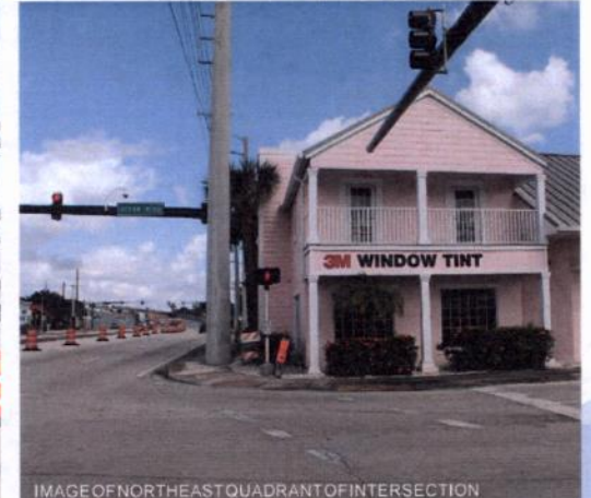
IMAGE OF NORTHEAST QUADRANT OF INTERSECTION
