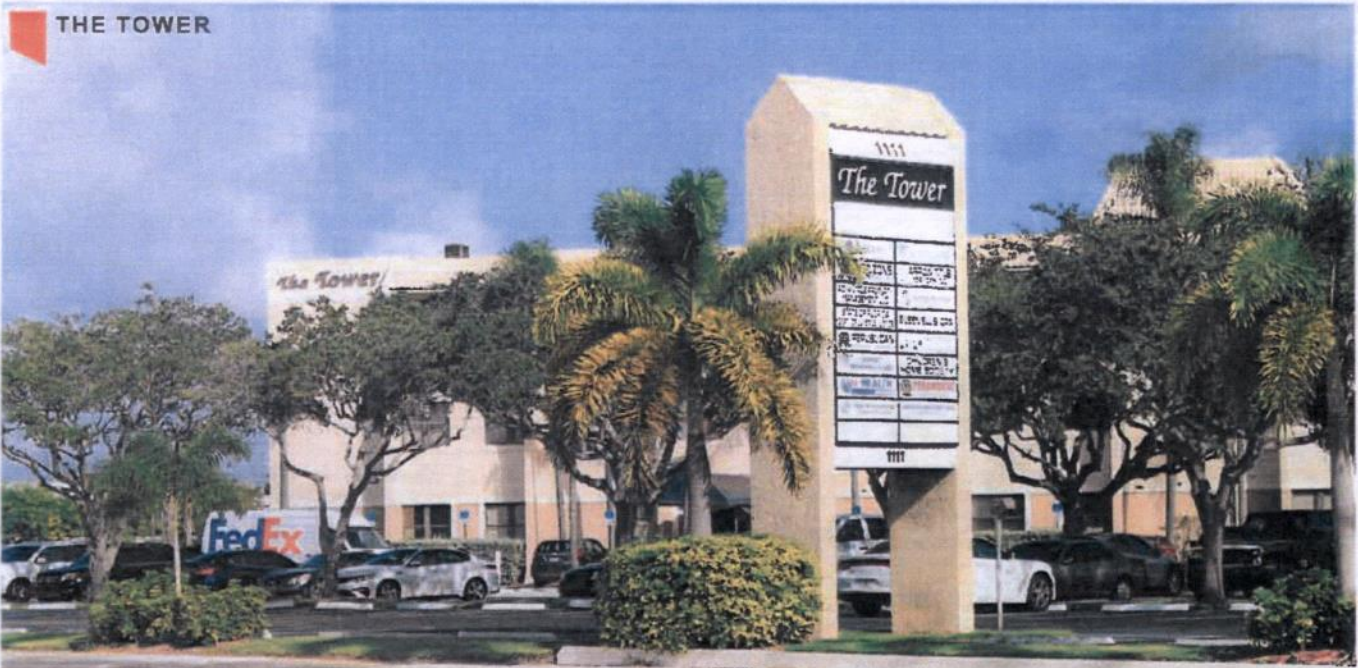
Figure 102 Image of site from Southeast Federal Highway.
