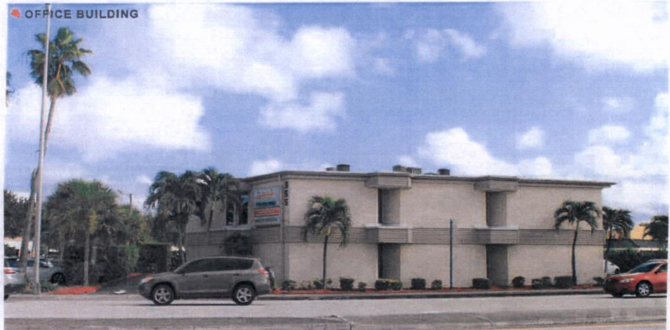
Figure 122 Image of site from Southeast Federal Highway.
