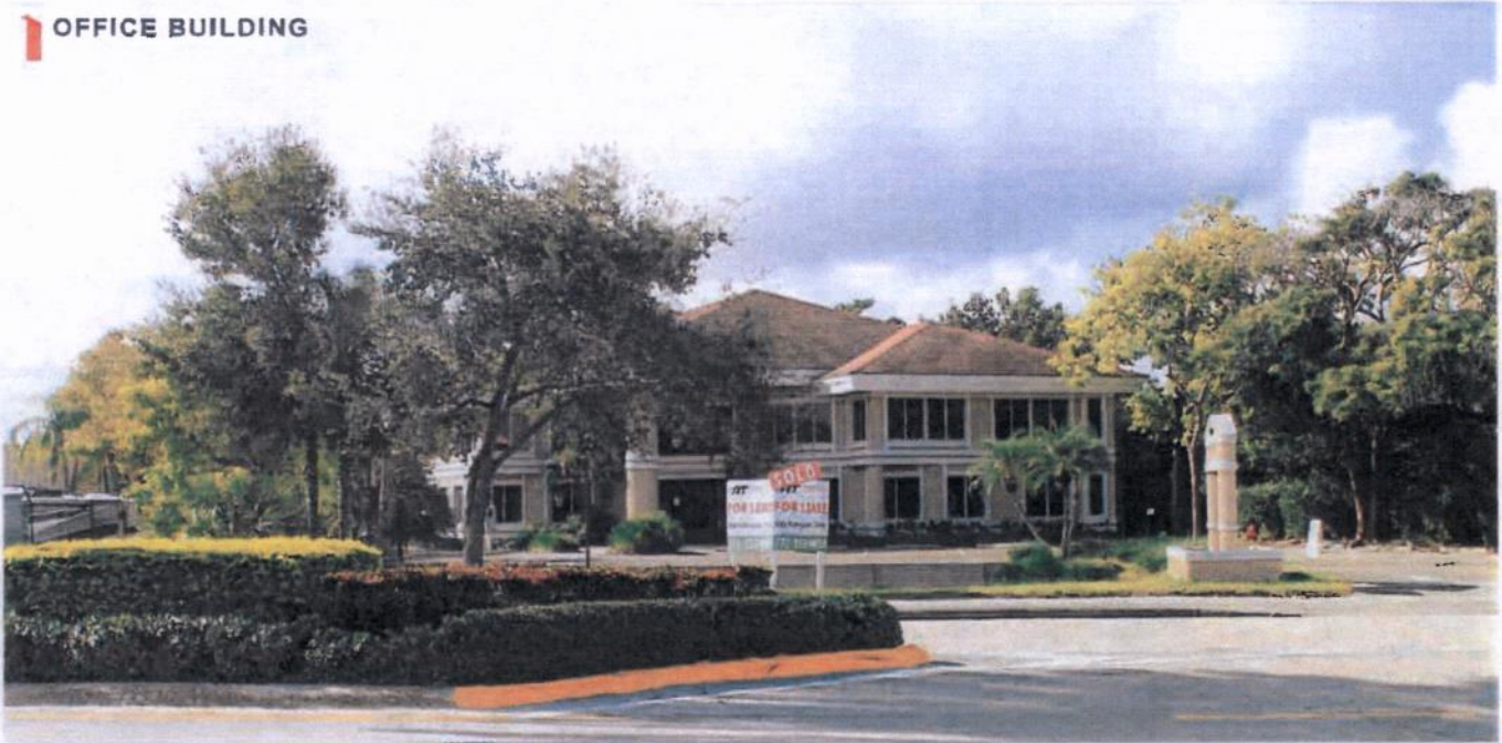
Figure 52 Image of site from Southeast Federal Highway.
