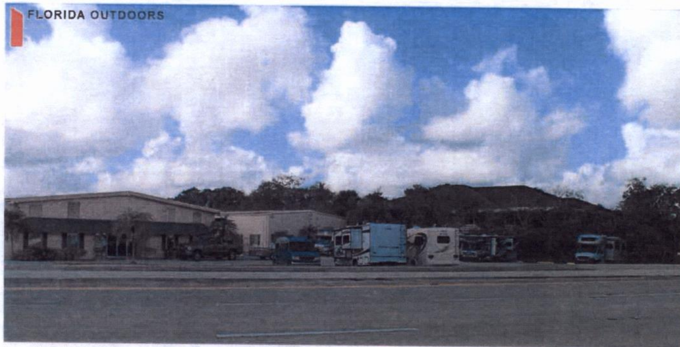
Figure 80 Image of site from Southeast Federal Highway.
